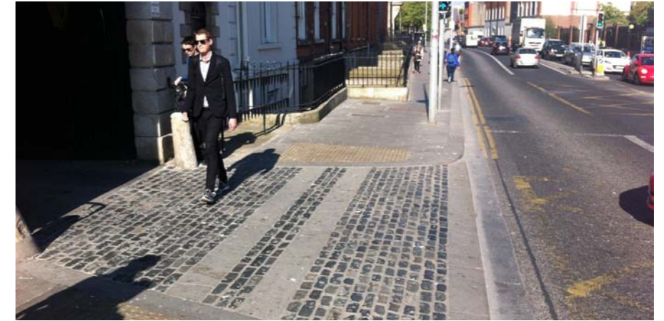
Pavement level crossing utilising heritage setts, St. James Street
