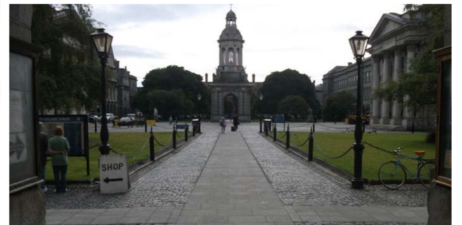
Smooth stone flags set into Heritage cobbles for Universal Access, Trinity College, Dublin
