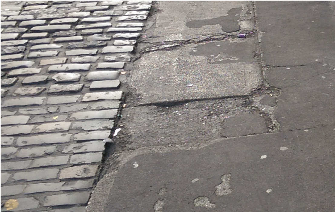
Poor reinstatements - bitumen replacing heritage setts
