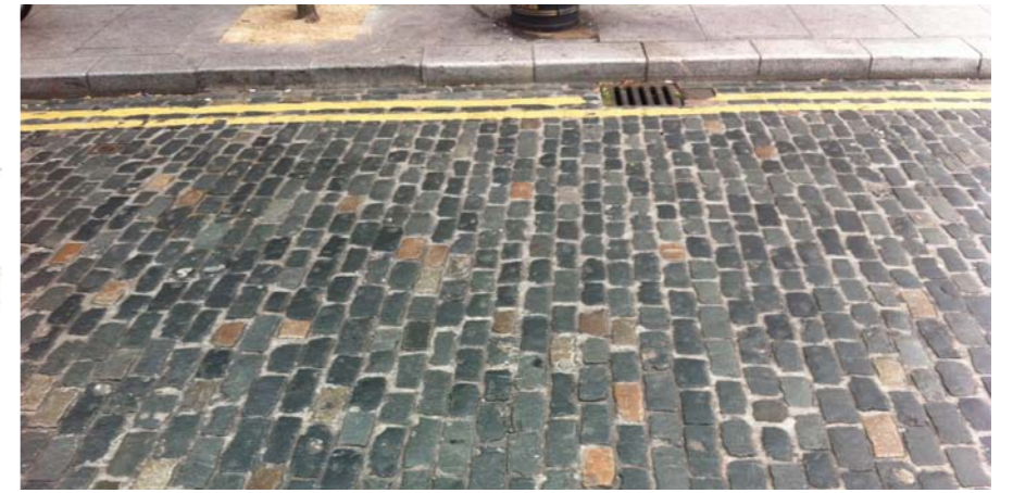
Heritage setts restored and relaid, narrower joint, cement/mortar joint.
