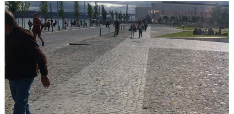
Heritage cobbles with saw cut top to create cycle-lane, Ribeira das Naus, Lisbon
