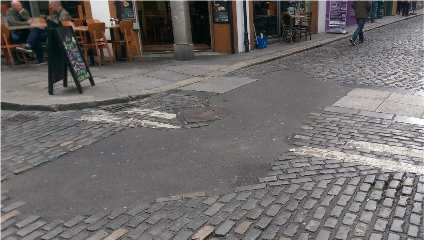
Poor reinstatements - bitumen replacing heritage setts
