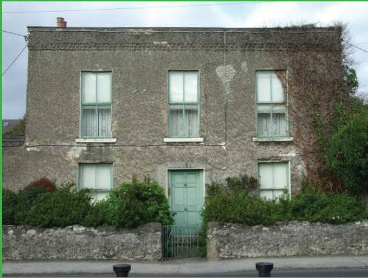
Fig. 23: Historic render and timber sash windows
