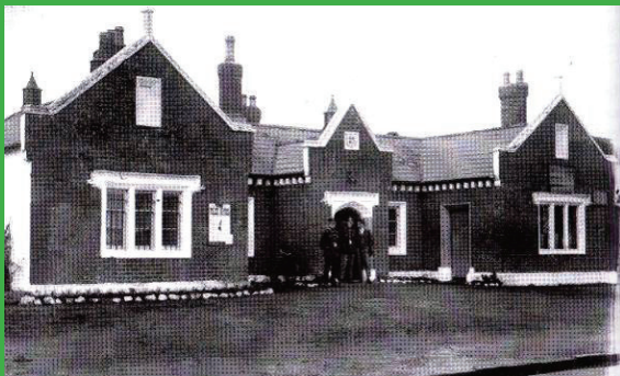
Fig. 14: Old Police Barracks, 1928/29
