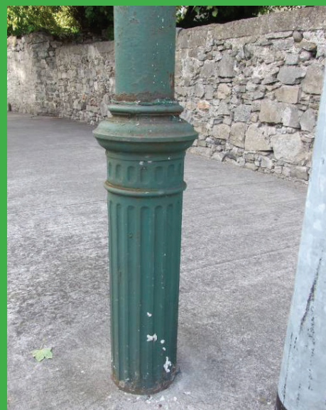
Fig. 70: Detail of historic lighting mast
