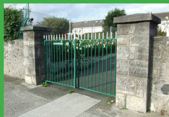
Fig. 28: Stone piers and metal gates to a dwelling
