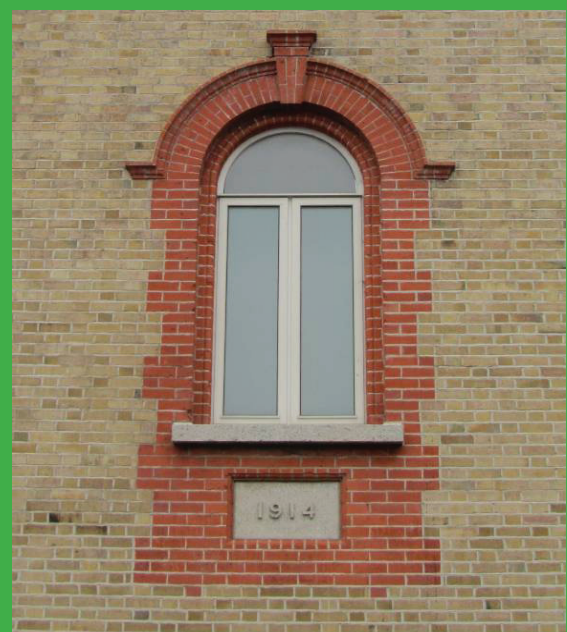
Fig. 22: Brick façade of former national school
