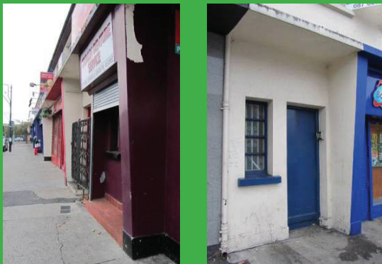
Fig. 59: Detail of terrace shop fronts
