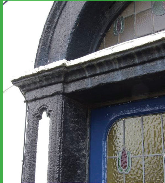
Fig. 25: Decorative stonework to the entrance of the former Glebe House
