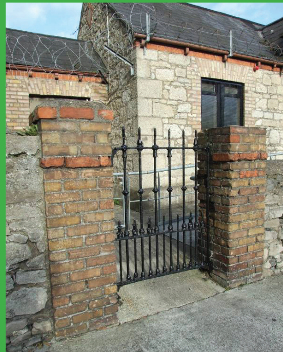
Fig. 27: Entrance to former school
