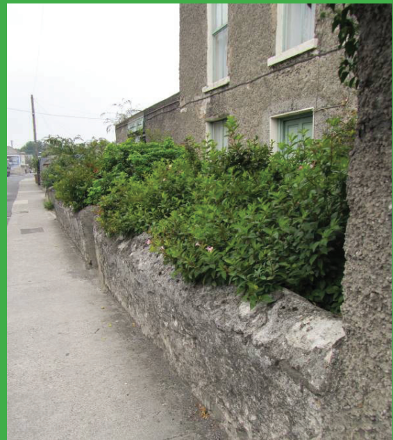
Fig. 31: Rendered rubble stone wall and piers
