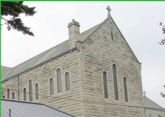
Fig. 24: Quarry faced stone and dressed stonework to the Catholic church
