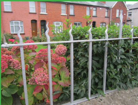
Fig. 29: Metal railings on plinth walls to row houses
