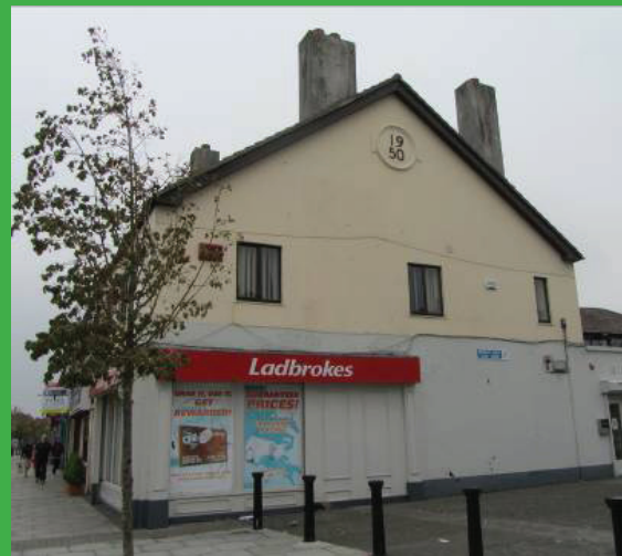
Fig. 63: Gable of terrace with '1950' date plaque
