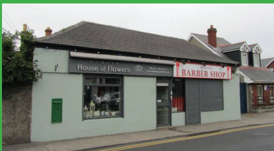
Fig. 56: Former post office
