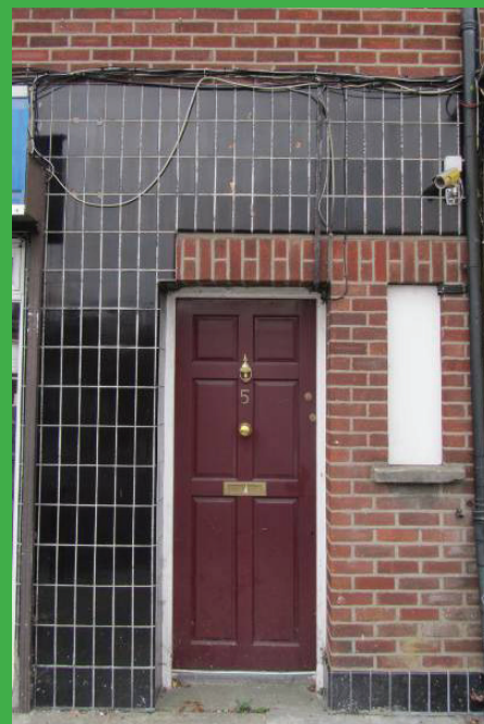
Fig. 61: Detail of entrance in terrace to upper floor
