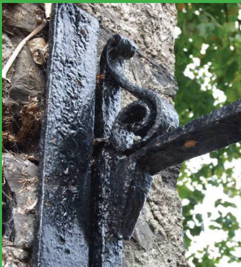
Fig. 34: Detail of metal gates to grounds of former St. Mary's church
