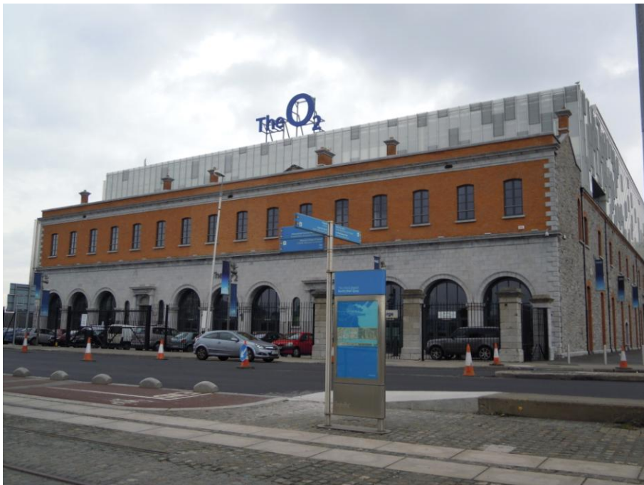
Former Goods Depot – North Wall Quay –(The O2)
