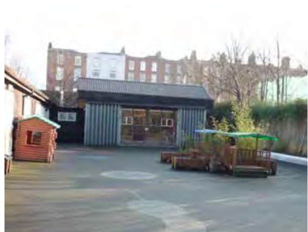
Fig. 31 View of nursery extension from the west.
