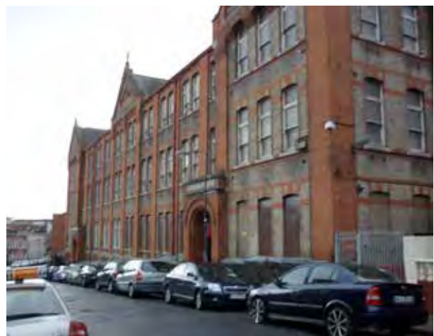
Fig. 86 View of former convent school at Rutland Street Lower.
