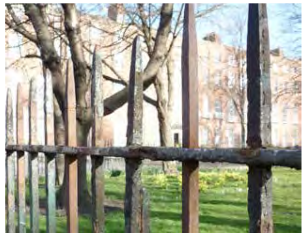
Fig. 35 Detail of section of railing repaired using mild steel.
