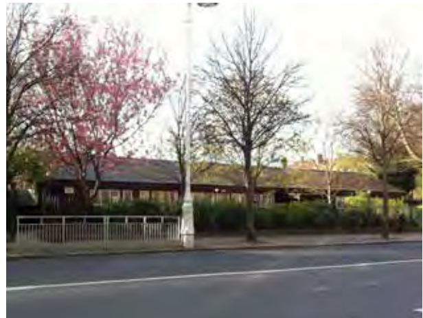
Fig. 30 View of nursery from Mountjoy Square North.
