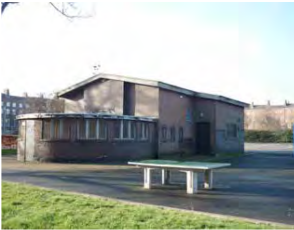
Fig. 28 View of community centre from north-east.
