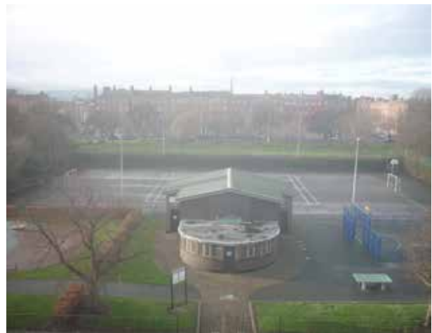
Fig.27 View of community centre from upper floor of no. 25.
