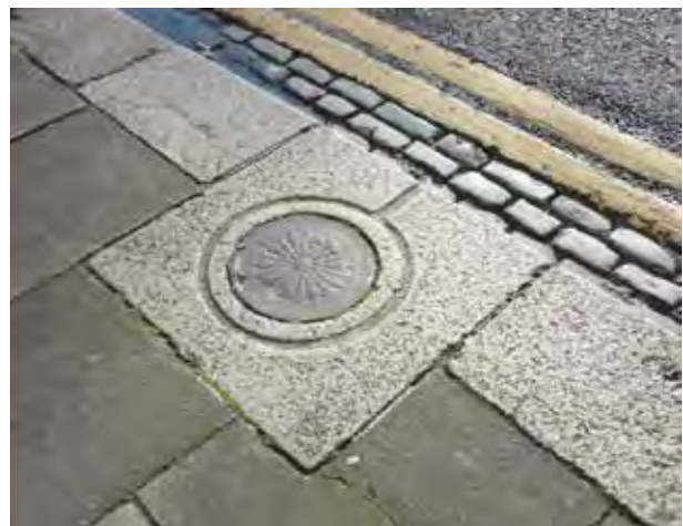
Fig. 40 Detail of coal hole cover set into granite kerb stone surround.
