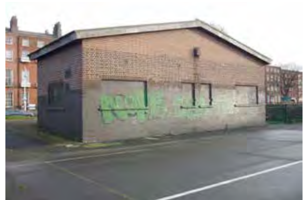
Fig. 63 View of west side of the Community Centre.
