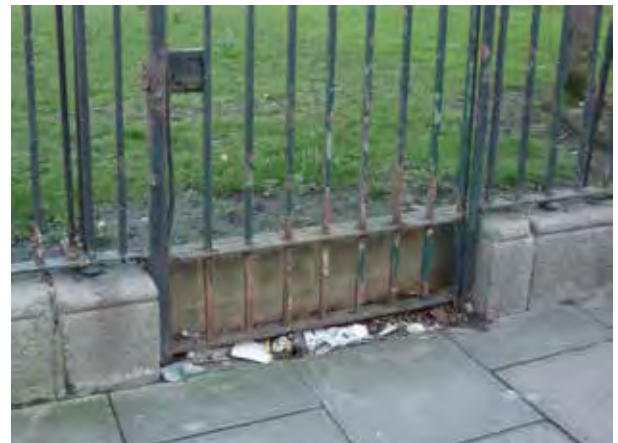
Fig. 34 Detail of infilled gate to removed public toilets.
