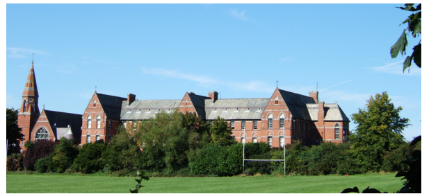
Fig.17: View of front elevation of O'Brien Institute
