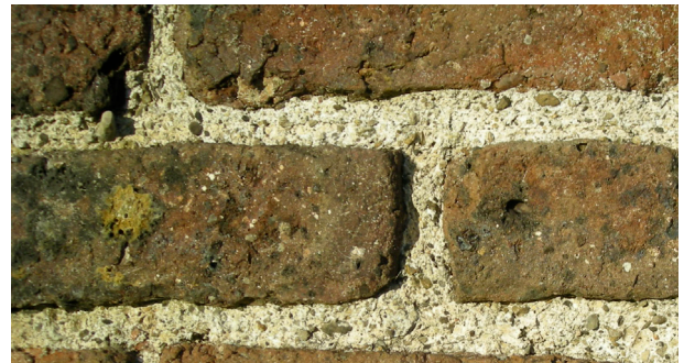
Fig.21: Detail of brick and lime mortar from boundary wall
