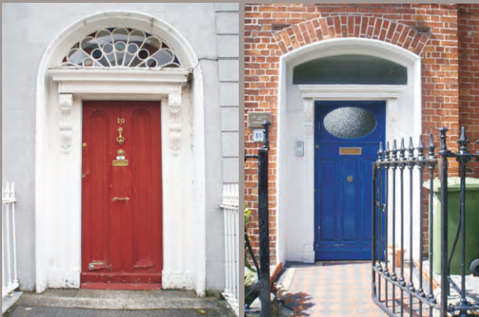
Mid 19 th century door on Newgrove Avenue and a mid 19 th century door surround with an attractive replacement early 20 th century door on Gilford Road.
