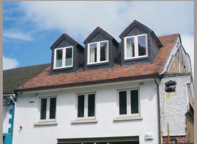
20 th century red tile roof with dormer windows
