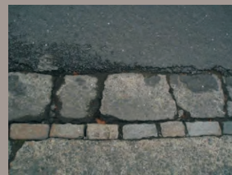
Stone gully sets and curved granite kerbing.
