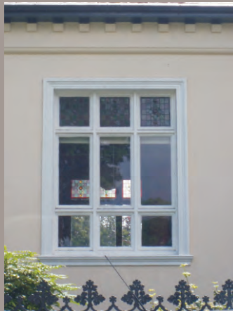
Examples of two windows on Sandymount Square: Ryan's Pub with replacement timber casement window and Sandymount Castle timber casement window with stained glass panes.
