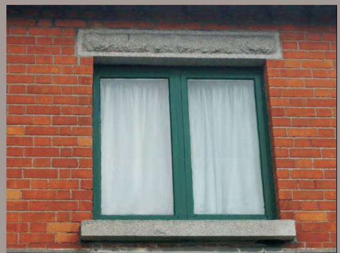
Ground and first floor timber casements from St James Terrace with fine granite lintel and sill.
