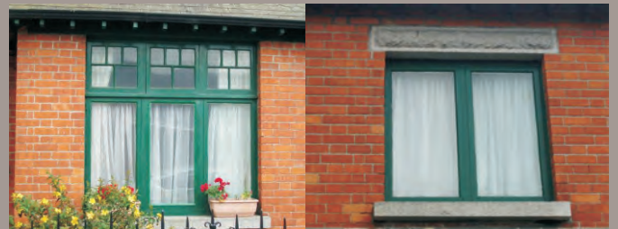
Original timber casement windows with granite dressing.
