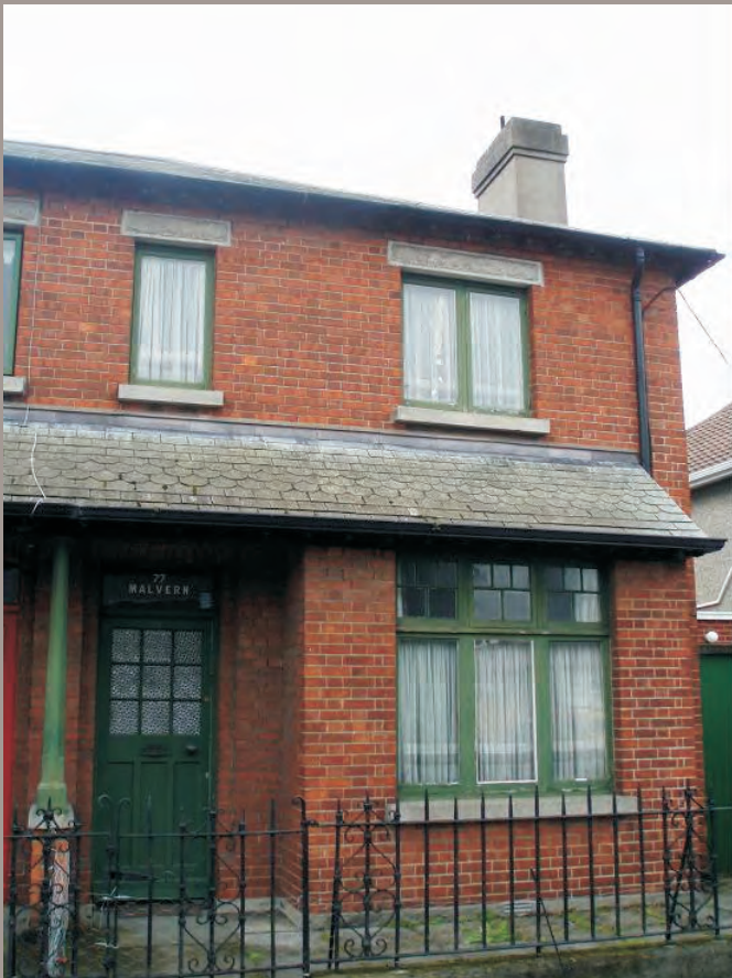
End of terrace house retaining all the original architectural detailing.
