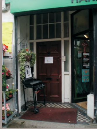
Recessed first floor entrance with flat panelled timber door and large overlight with the original tiling to the entrance porch on Sandymount Road.
