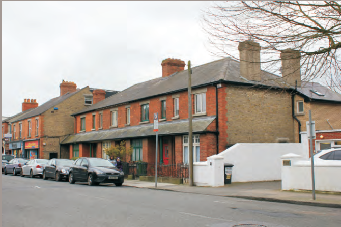
View of slate roofs along St James Terrace Sandymount Road.
