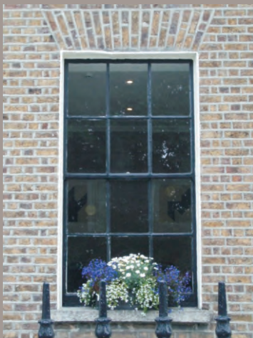
Six-over-six timber sash window without horns with early glass
