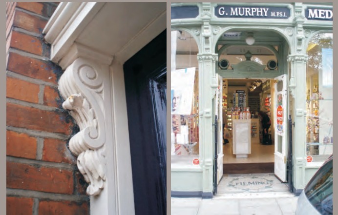
Examples of carved timber detailing is also found around door surrounds. For example this console bracket on Newgrove Avenue and on Murphy's Shopfront on Sandymount Green.
