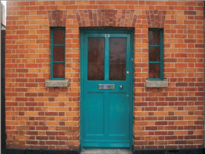
Early twentieth century timber and glazed door flanked by fixed pane sidelights having granite sills.
