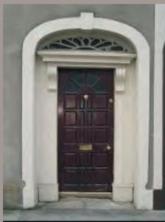
One of a pair of recessed entrance doors with the original surround and compressed leaded fanlight.
