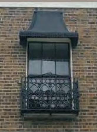
Decorative canopy and cast-iron balconette add immense architectural appeal to a sash window.
