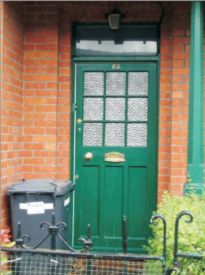
Original timber and glazed door with early door furniture.
