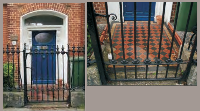
Original doorcase and early twentieth century door. The railed front site has polychromatic terra cotta tiles.
