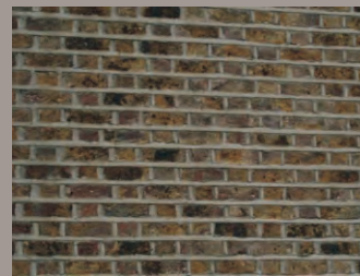
Nineteenth century man made yellow brick laid in a Flemish bond with heavy cement strap pointing.
