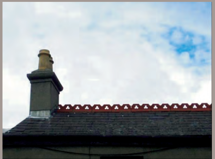
Original natural slates and terracotta ridge comb on Seafort Avenue.
