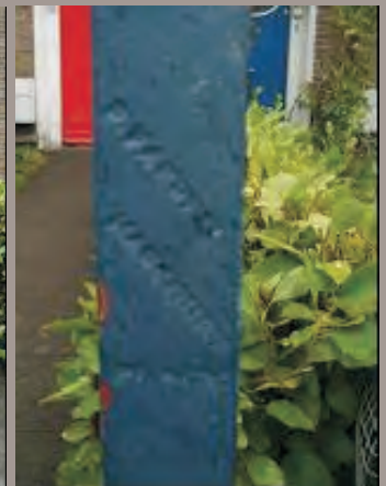
Wrought and cast-iron railings with anthemion detail and manufactures mark on the slam bar from a foundry on Harcourt Place, possibly D.Farden.
