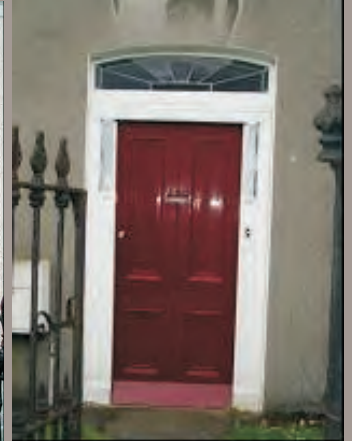
Compressed segmental-headed doorcase with leaded fanlight and timber flat panelled entrance door with central finial.
