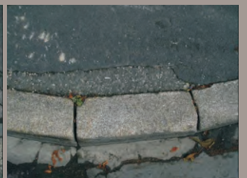
Stone gully sets and curved granite kerbing.
