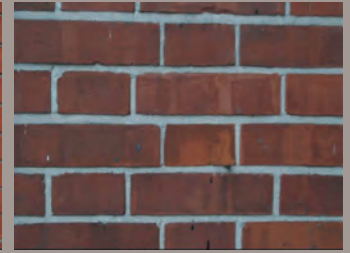
Machined red brick laid in Flemish bond with narrow cement mortar pointing from different brickyards on Gilford Road.
