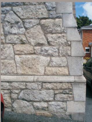
Rock-faced granite wall to church on Newgrove Avenue with cut stone quoins.
