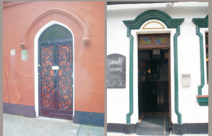
Two doorways on the southeast and north end of Sandymount Green displaying decorative rendered or stucco detailing.
