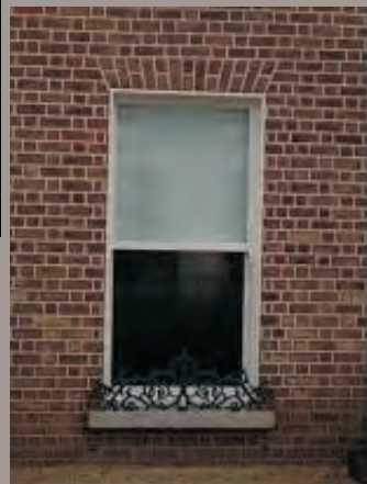
Cast-iron vignette on the ground floor cill designed to secure a window box.
