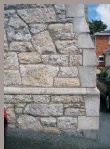
Detail of granite wall
