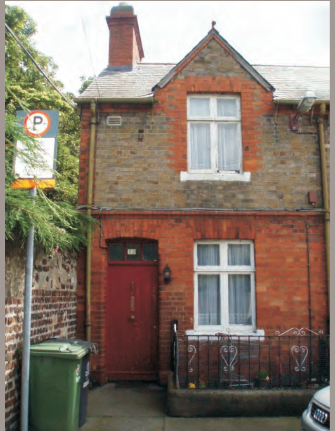
Polychromatic brick, original joinery and roof slates make for attractive architectural detailing.
