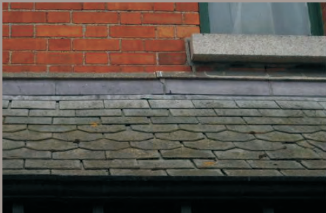
Detail of fish scale tiles on the porch of St James Terrace.
