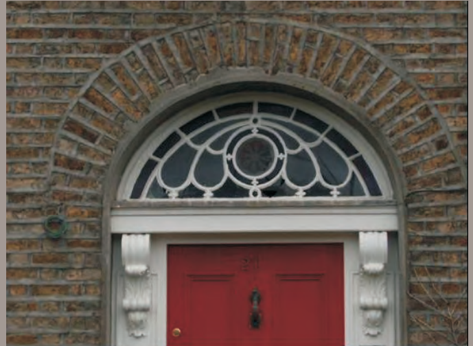
Teardrop led fanlight with attractive Victorian coloured glass.
