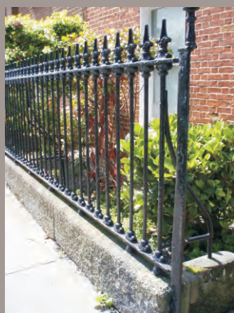
Examples of cast-iron railings surmounting granite plinth walls on Newgrove Avenue and Gilford Road.
