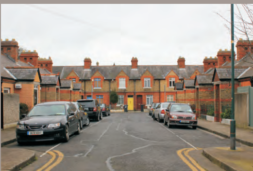
General view of single-storey and two-storey cottages of Seafort Avenue.
