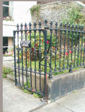
Wrought-iron railings with cast-iron decoration with vehicle gate.
