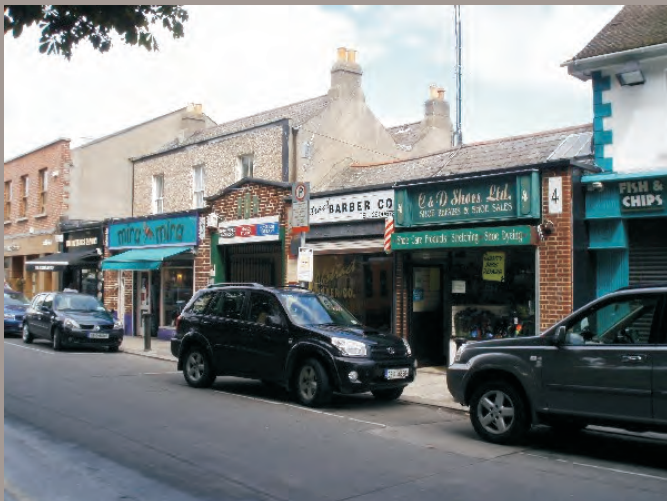
1940's shopfront on NE side of Sandymount Green
