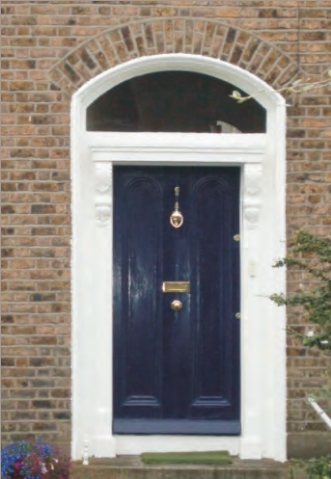
Late nineteenth century door with elongated flat panels with carved timber corbels supporting the segmental-headed fanlight.
