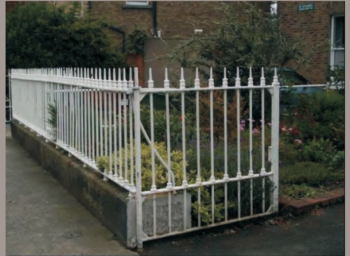
Wrought-iron railings with cast-iron decoration with vehicle gate.
