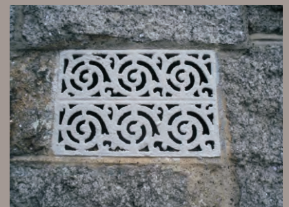
Metal vent to side
