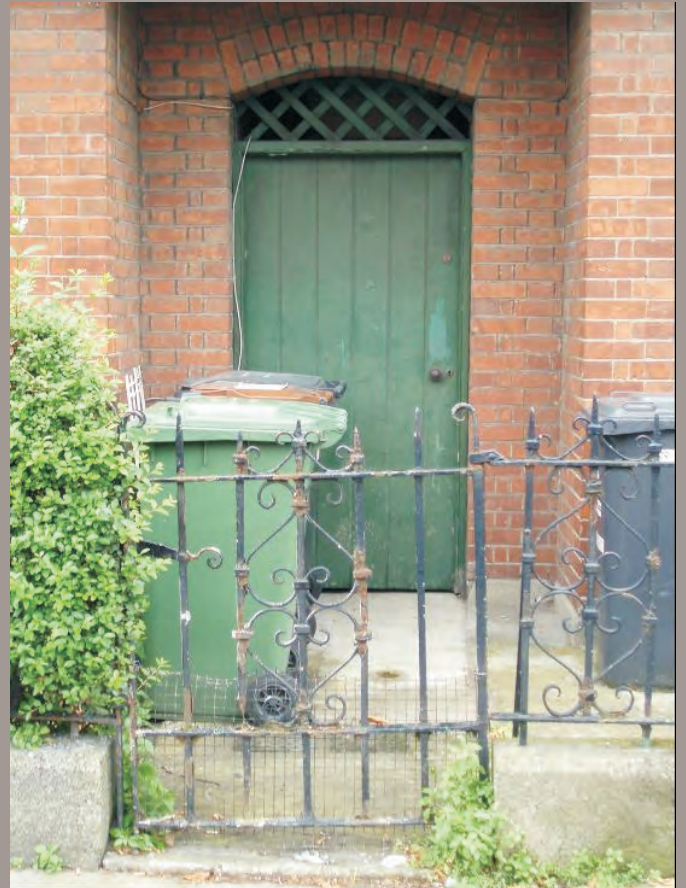
Original tongued and grooved ginnell alleyway affording rear access to the rear site of the middle houses in the terrace.
