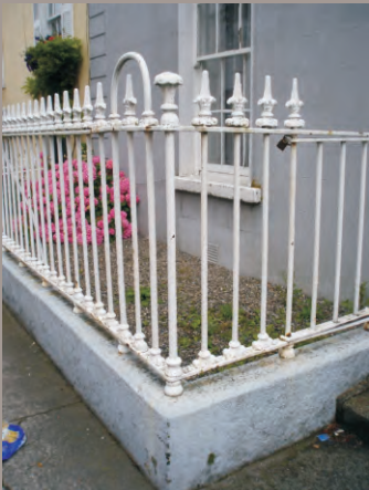
Examples of cast-iron railings surmounting granite plinth walls on Newgrove Avenue and Gilford Road.
