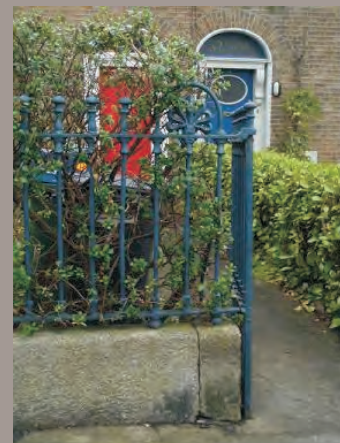
Wrought and cast-iron railings with anthemion detail and manufactures mark on the slam bar from a foundry on Harcourt Place, possibly D.Farden.
