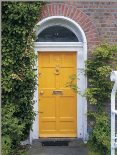
Mid to late 19 th century doors on Newgrove Avenue displaying their original timber panelled doors which are well maintained.
