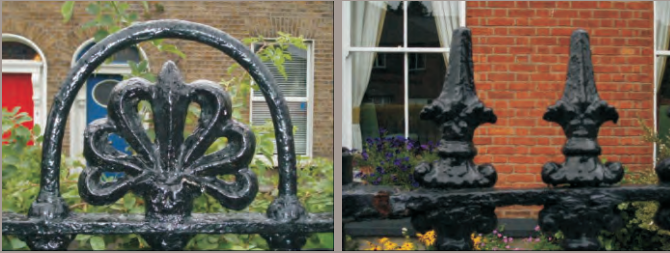
Cast-iron finial details on various railings.
