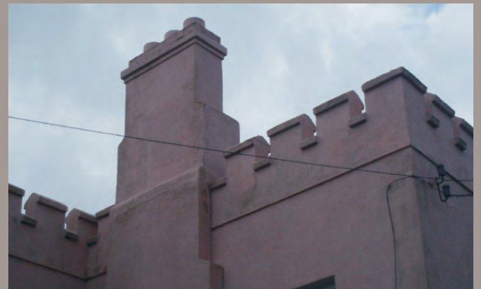
Battlemented parapet to house on southeast side of Sandymount Green
