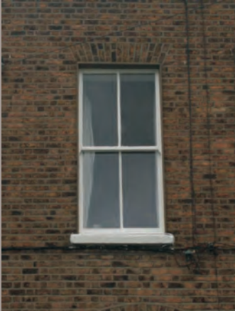
Two-over-two timber sash window with convex horns on Claremount Road.
