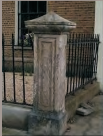
Capped corner pillar and simple wrought iron railing on Sandymount Green.
