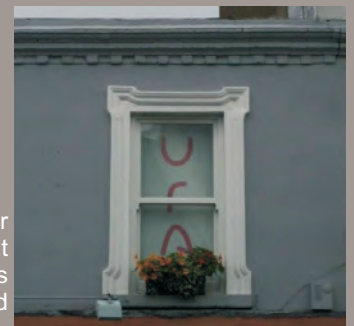
Ground and first floor timber casements from St James Terrace with fine granite lintel and sill.
