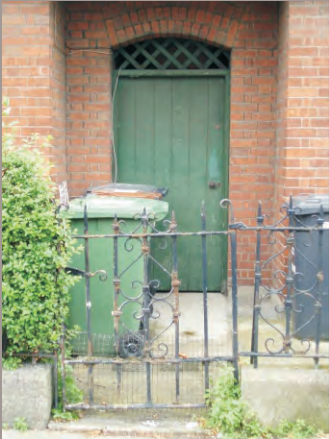
Twentieth century railing on a granite plinth and gate on St James Terrace.
