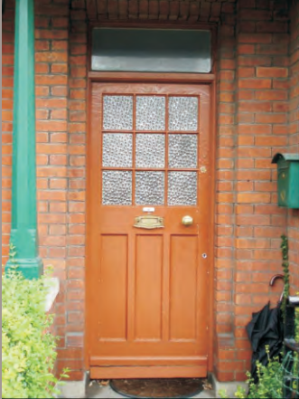
Twentieth century glazed and panelled door with early door furniture on St James Terrace.
