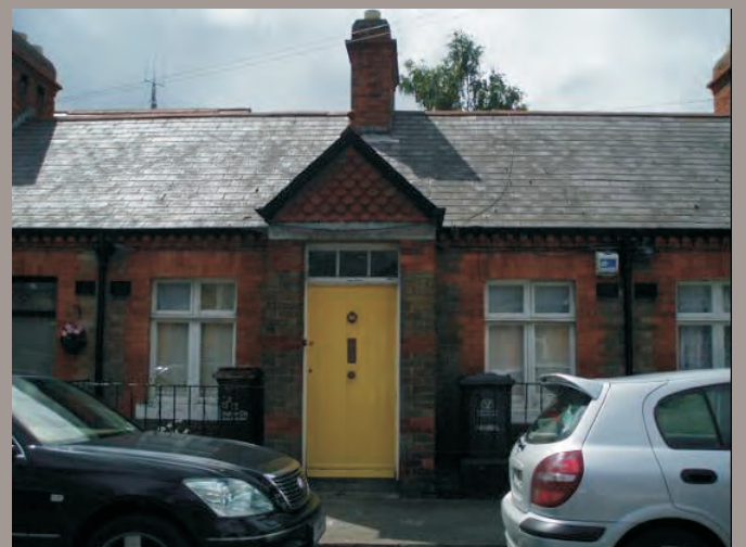
Single-storey cottages with terra cotta detailing to the porch, brick corbels and original joinery.
