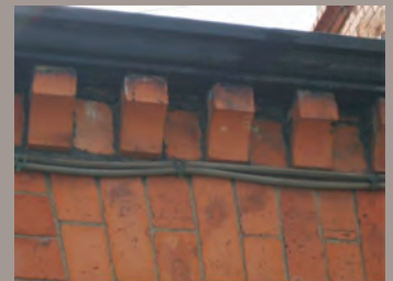
Machined brick corbels supporting an exposed cast-iron gutter on Seafort Villas.
