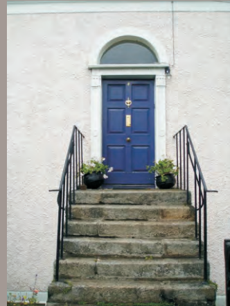
Fluted doorcase with round-headed fanlight with a tall flight of granite steps with wrought iron railings. This raised entrance door is not the typical entrance door in the village.
