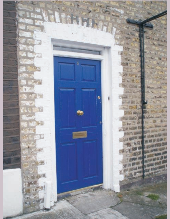
Replacement front door
