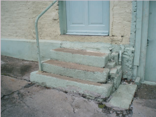
Granite steps at Temple Place
