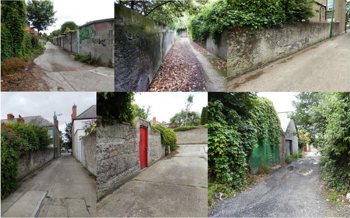
Views of rear laneways: Most historic rear walls no longer survive. One section of rubble calp limestone wall was identified on a side laneway boundary wall to 77 Hollybrook Road. The side boundary wall to 39 Hollybrook Road is constructed of brick. Remaining original walls are largely of early mass concrete construction.
