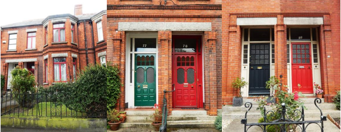
Pre war (circa 1911-1914) houses constructed on eastern side of south end of street display decorative terracotta detailing and attractive recessed doors.
