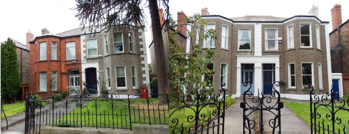
Most of the houses on the street are composed of semi-detached pairs with hipped roofs, tall chimneys to side elevations and bay windows. Front doors are set in recessed porches. Overtime the some of the original red brick facades have been subject to later early to mid 20 th century decorative render treatments.
