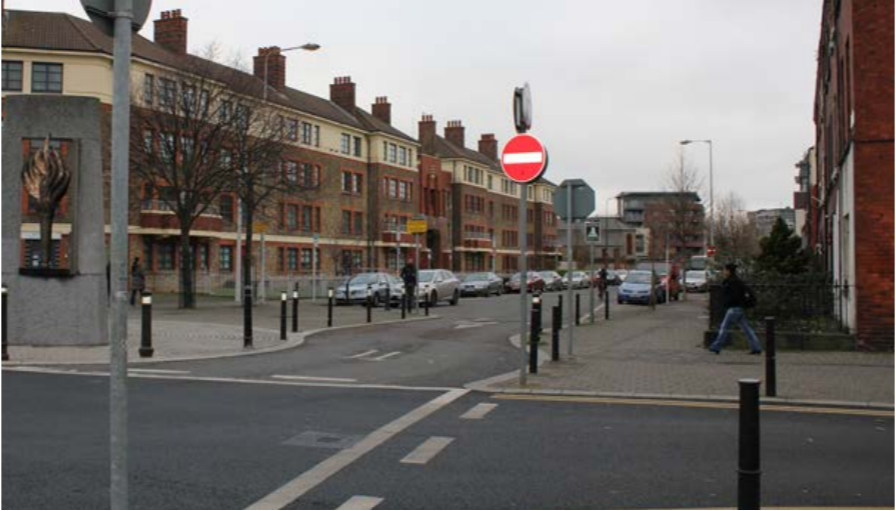
Existing: View from Sean MacDermott Street showing traffic calming carriageway narrowing
