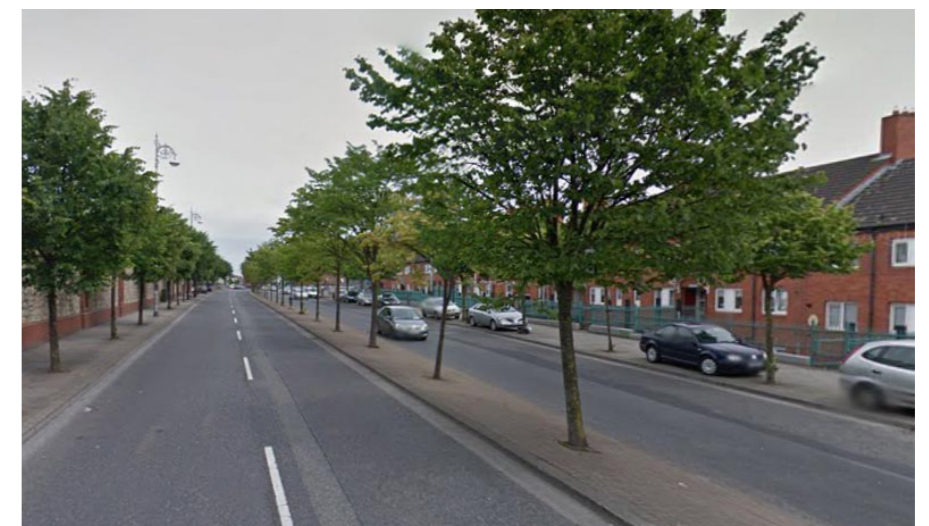
Existing: Central median strip on Summerhill
