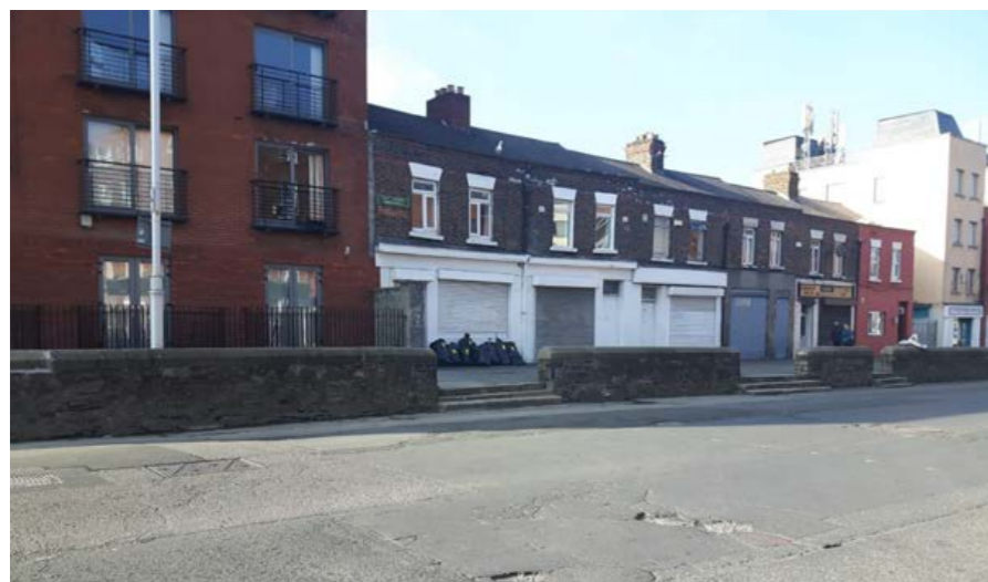
Existing: Stepped terrace and wall on Summerhill Parade
