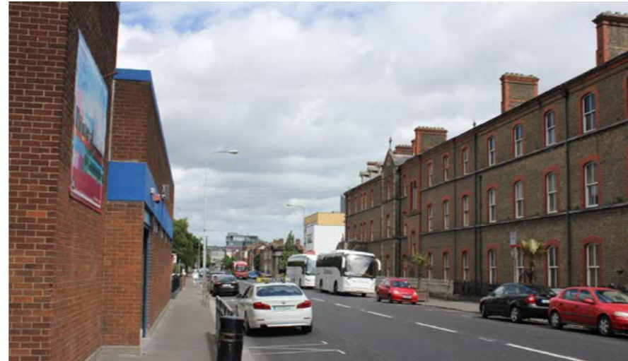
Existing: Public Swimming Pool with Magdalene Laundry Building opposite
