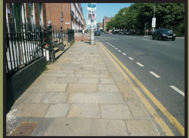
Figure 22 : Granite paving & kerb stones outside no. 54.
