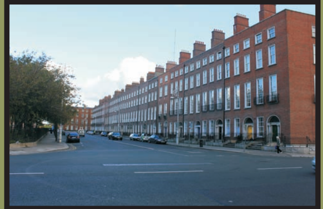
Local View 12 : Looking East On Mountjoy Square South
