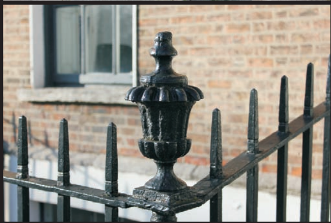
Figure 13: Cast Iron railings with plain finials and urn standard heads
