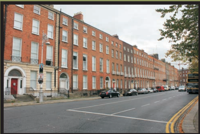
Local View 5 : Looking North East On Mountjoy Square North
