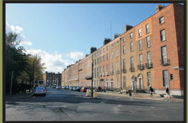
Local View 7 : Looking West On Mountjoy Square North
