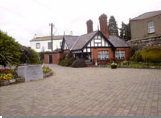
The Blessington Street Basin Entrance
