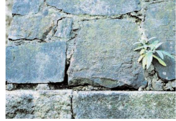
Plate 4 Open joints in the City Wall.
