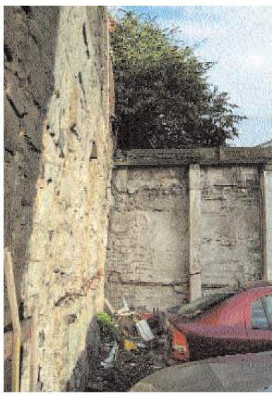
Plate 28 Structurally unstable standing remains at Ship Street Little.
