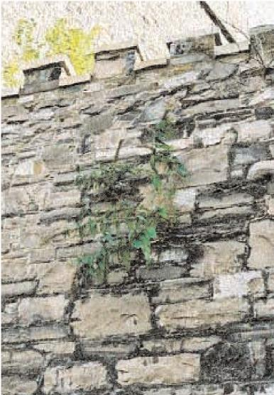
Plate 8 Sulphation of mortar.
