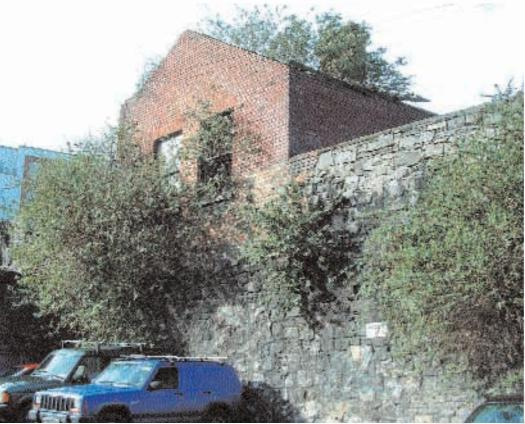
Plate 26 Original masonry and later interventions at Ship Street Little, near Werburgh Street.
