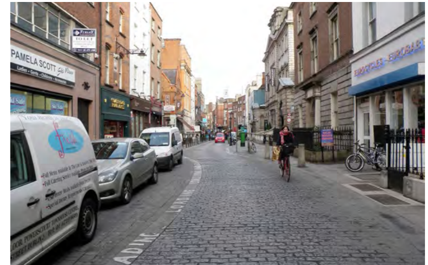
Existing Paved Carriageway
