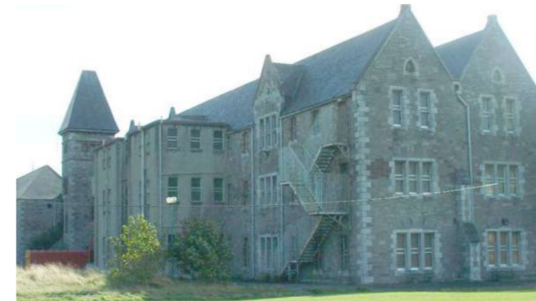
Exterior of Top House - View from North West
