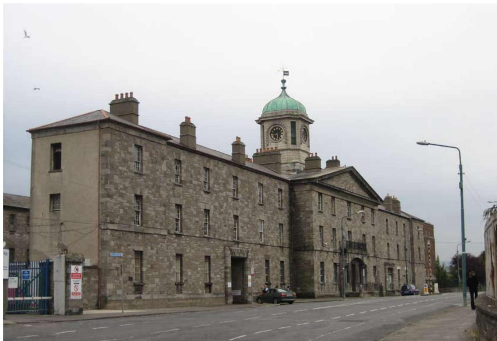
Exterior of Clock Tower Building (former penitentiary) – west elevation to Grangegorman Lower
