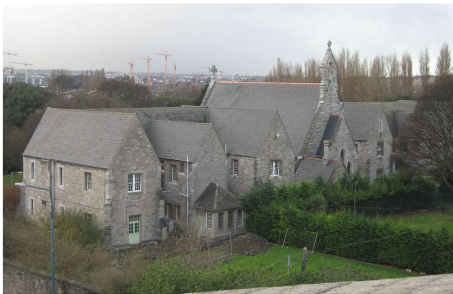
North elevation of female infirmary from roof of clock tower opposite—Catholic Church and male infirmary in background, together forming overall assembly of buildings
