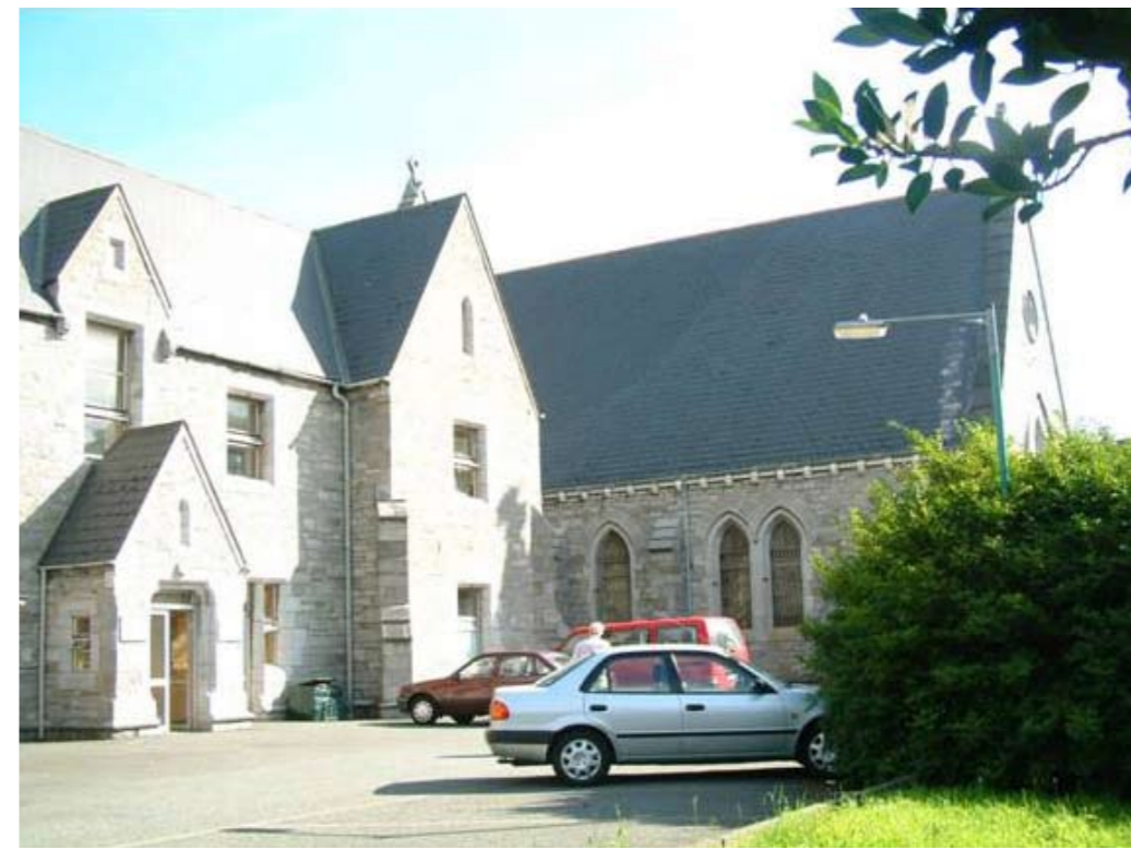
Exterior of male infirmary—south elevation with Catholic Church in background
