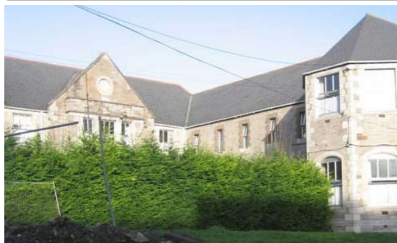
Exterior of female house—part of south elevation
