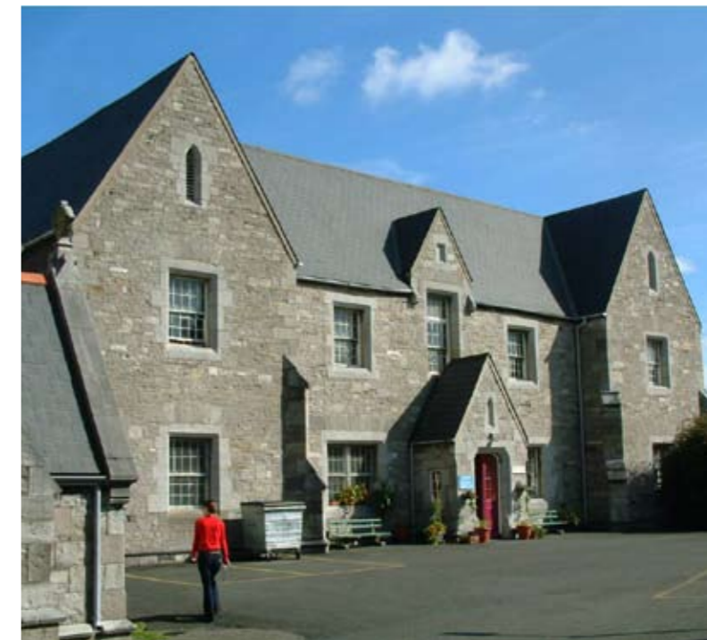
Exterior of female infirmary—south elevation
