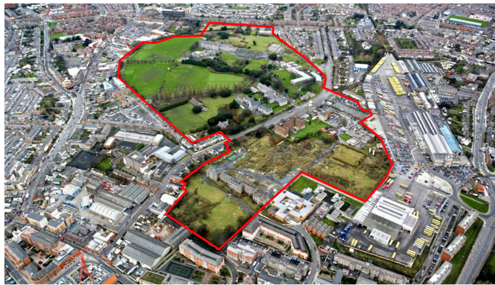
Aerial view of site from SE with Planning Scheme boundary
