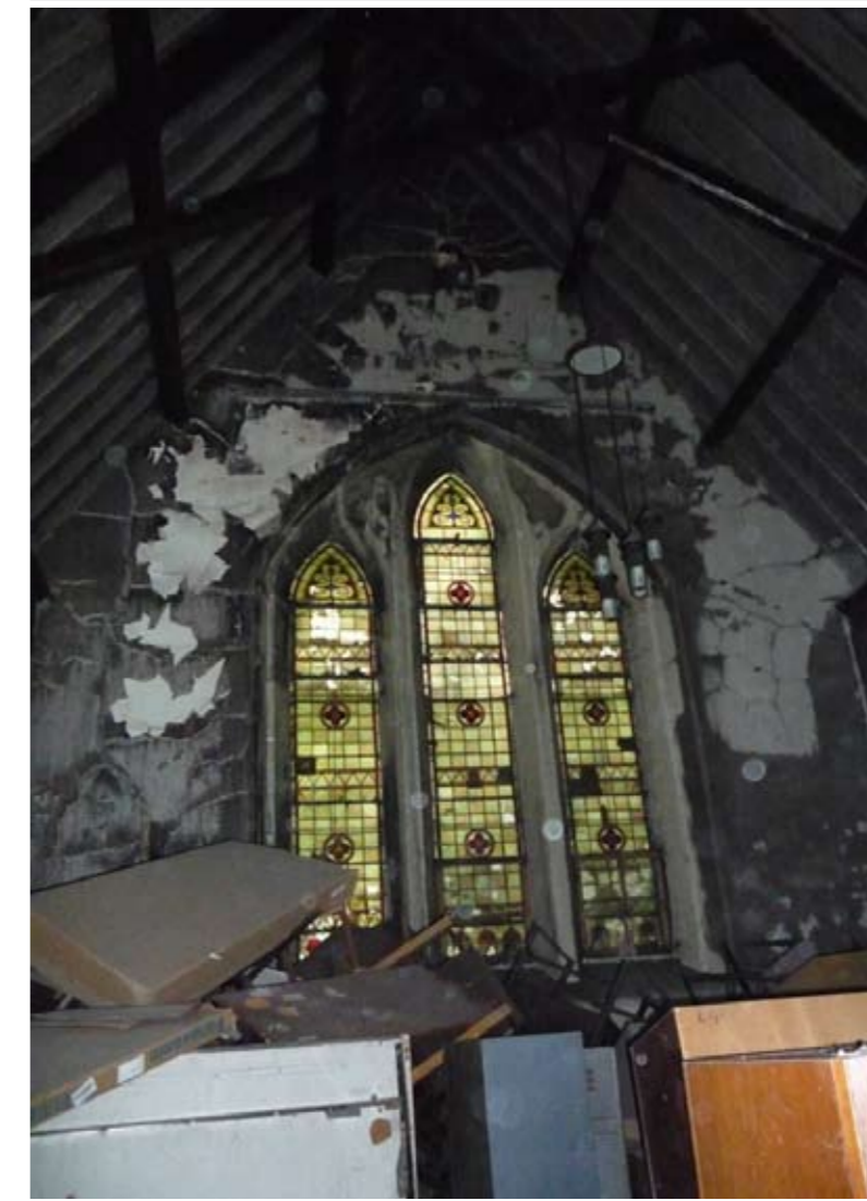
Interior of Church of Ireland chapel
