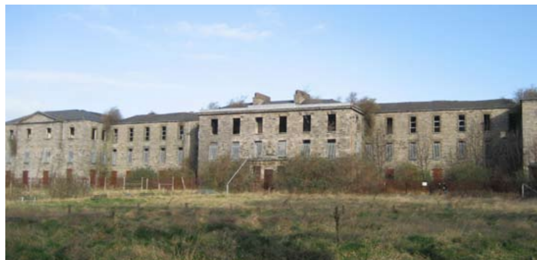
Exterior of Lower House (former lunatic asylum) – south (front) elevation
