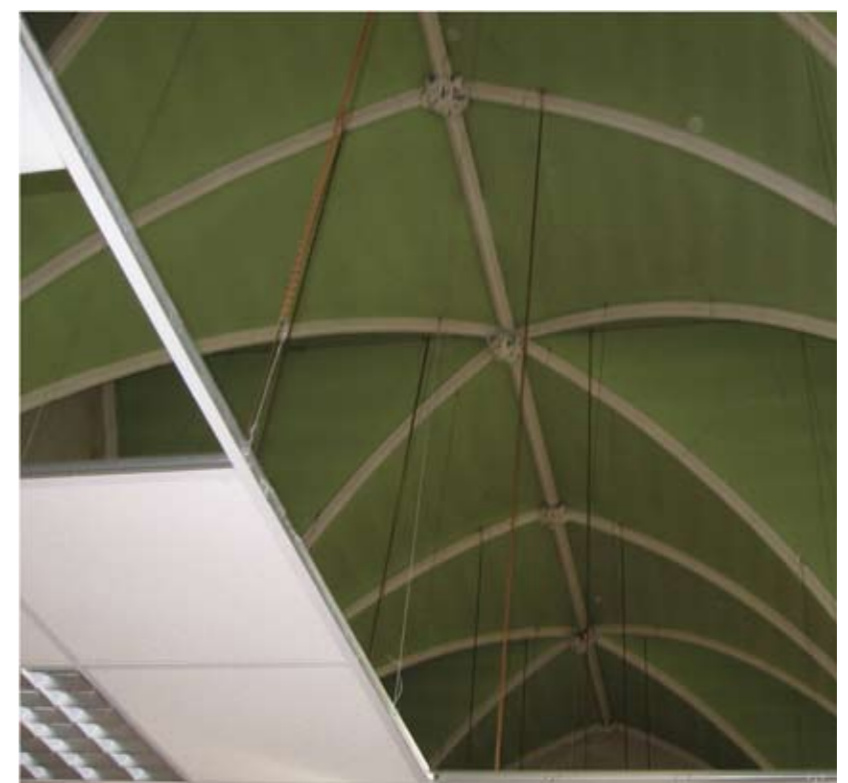
Rib vaulting to Chapel ceiling
