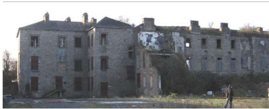
Exterior of Lower House (former lunatic asylum) – North (rear) elevation
