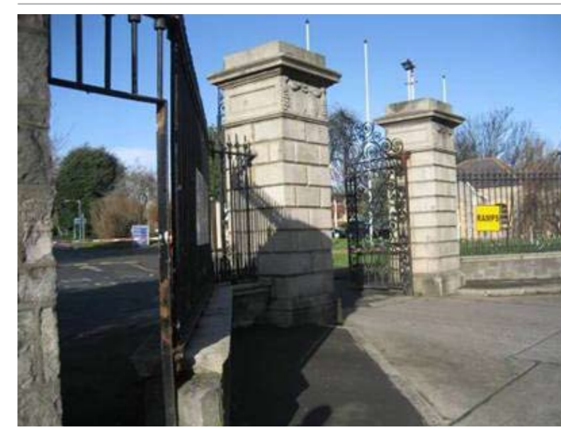
(above and left) Main Entrance gates and piers
