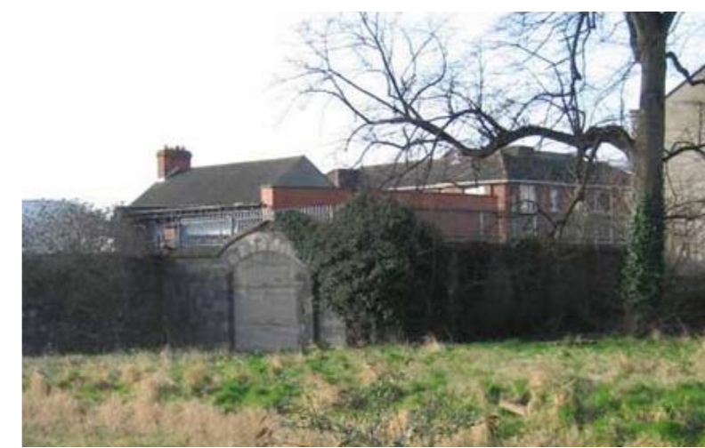
Arched entrance from Grangegorman lower to rear of surviving section of Lower House
