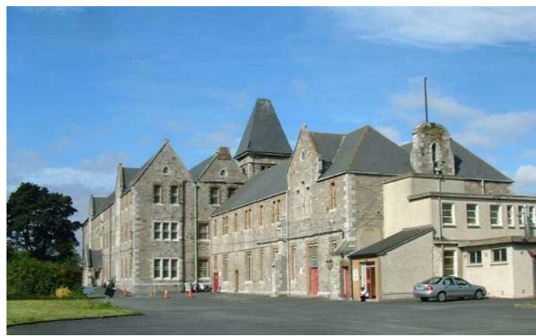
Exterior of top house—view from South East
