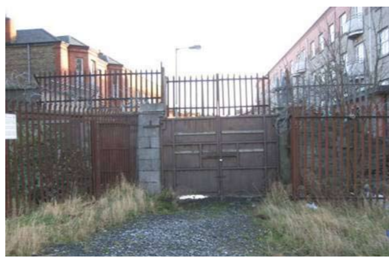
Access gate from Morning Star Avenue
