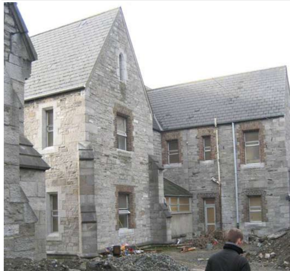
Exterior of male infirmary—part of north elevation
