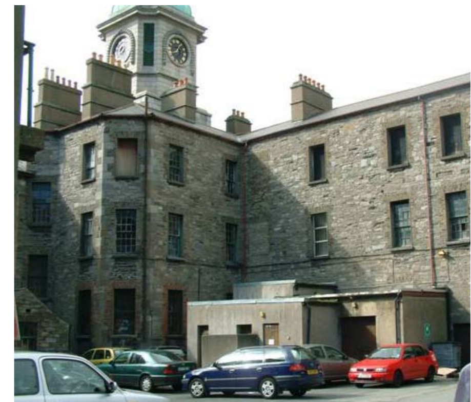
Exterior of Clock Tower Building (former penitentiary) – courtyard to east
