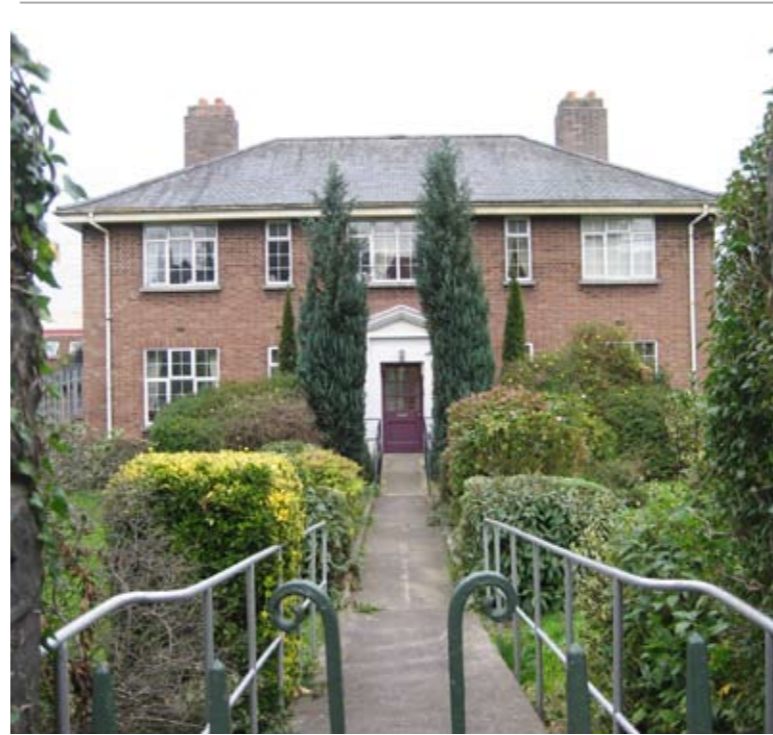
226 North Circular Road—former doctor's house. Nos. 228 & 230 are essentially identical structures.
