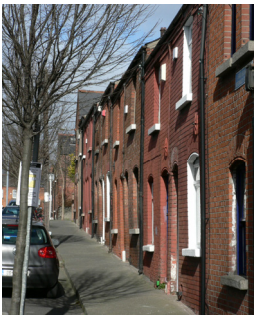
Stepped terraced housing on Reginald Street
