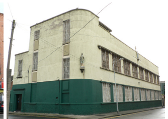
1930s Modernist former school building on Carman's Hall
