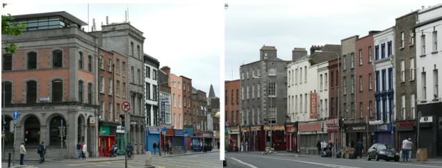
View of commercial buildings South side of Thomas Street looking west along Thomas Street approaching Meath Street.
