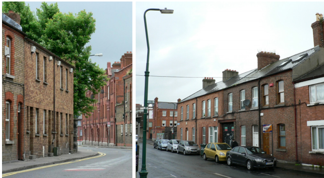
View along Thomas Court Victorian housing on Earl Street South showing cottage housing and the Guinness tenement block in the distance
