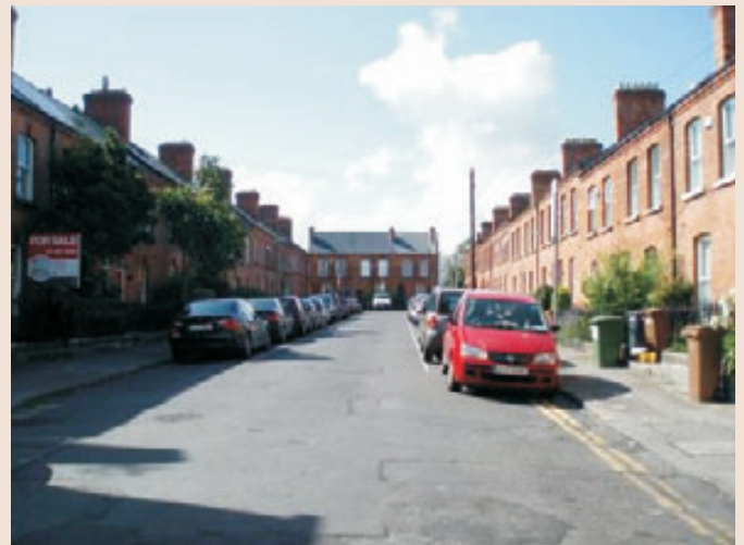
View of Streetscape Elmpark Avenue
