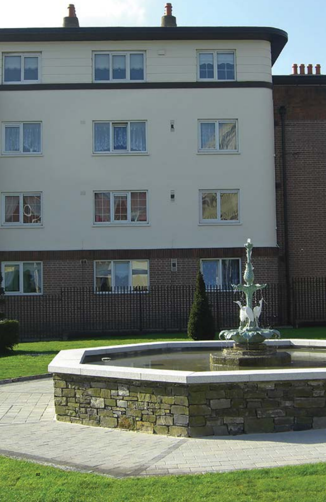
Chancery Street House and Chancery Park
