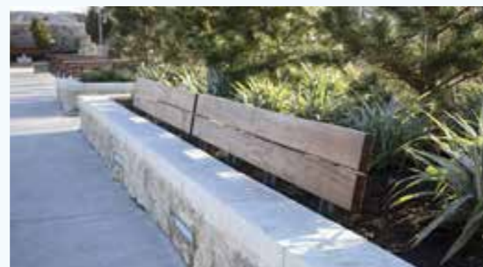
Example of seating walls with masonry top
