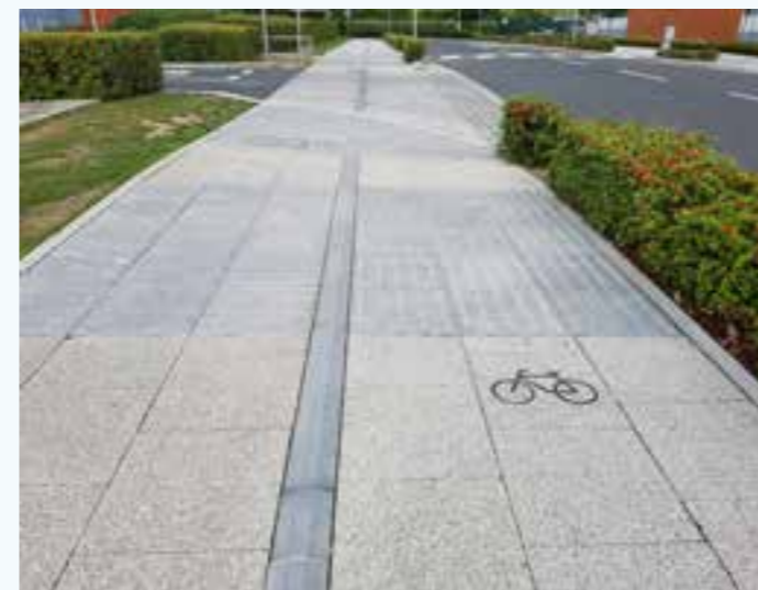
Example of a segregated cycle path integrated with paving and entrance treatments.
