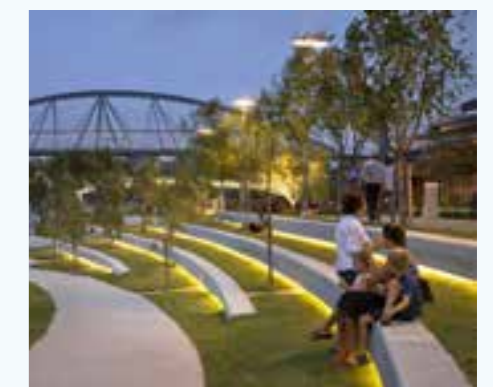
Example of lighting integrated into seating wall
