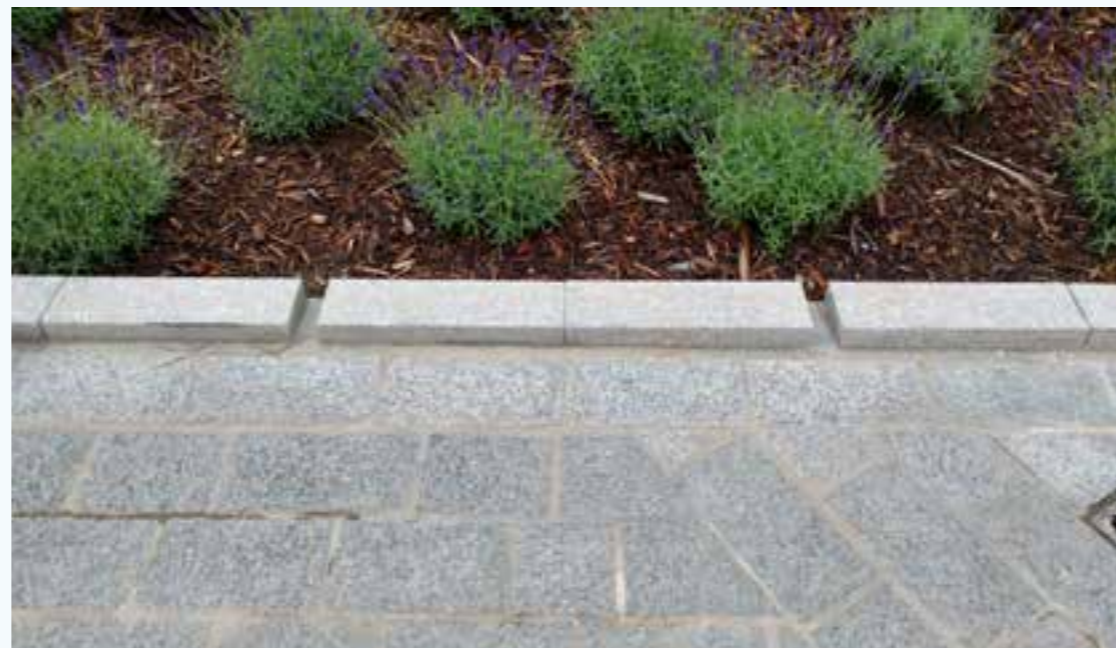
Surface water gully discharging directly into planting bed.
