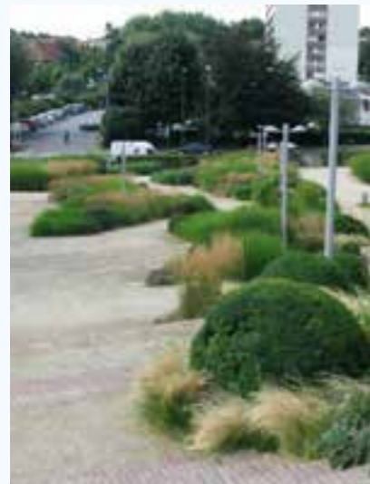
Figure A2.27. Hard surfacing draining directly into adjacent attenuating planting beds
