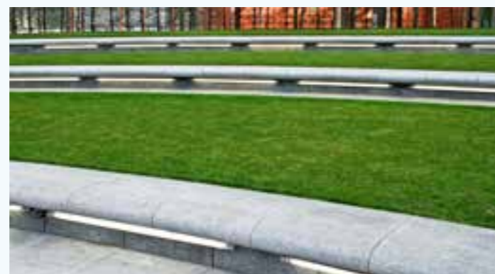
Example of grass terraces with granite retaining edges
