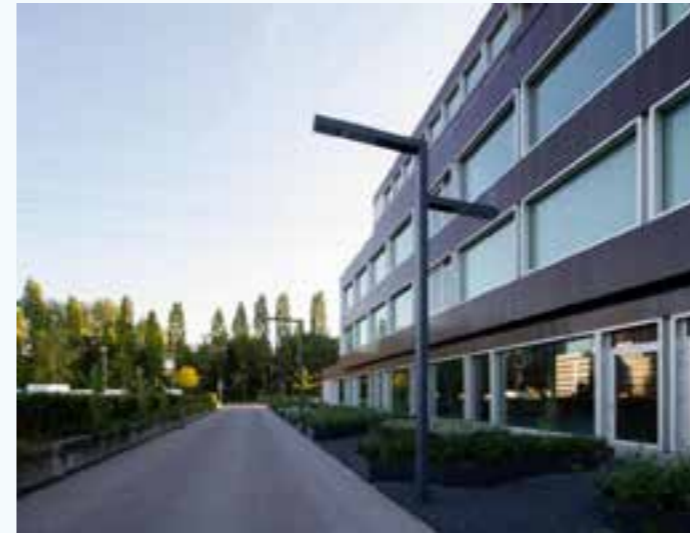
Example of street lighting with luminaries higher over the carriageway and lower over footway.
