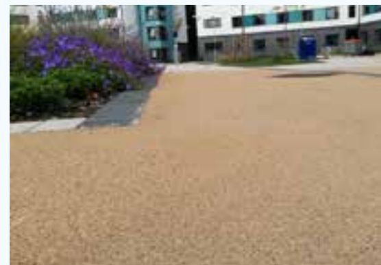
Bitumen macadam surface with coloured wearing course
