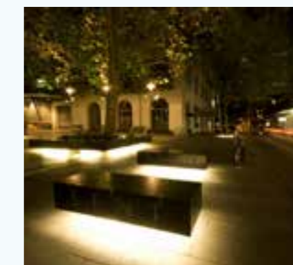
Lighting integrated into public realm seating
