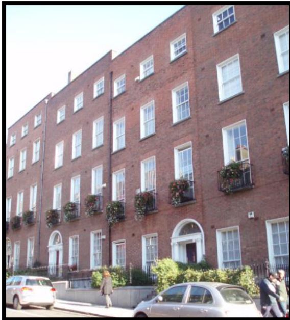
Figure 40 - Late 20th Century rebuilding of no's 29-34 with replica 18th Century style façade
