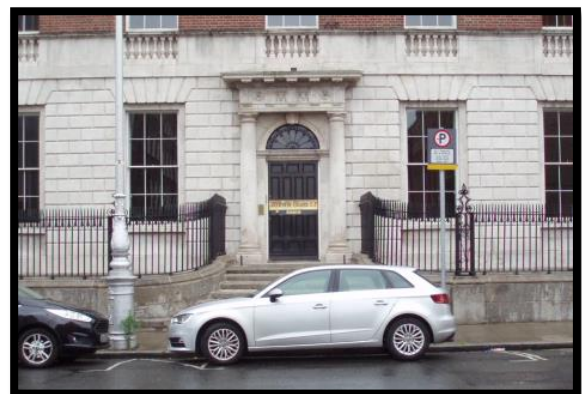
Figure 47 – No. 6 Denmark Street Great – splayed granite stepped entrance to 18th Century townhouse
