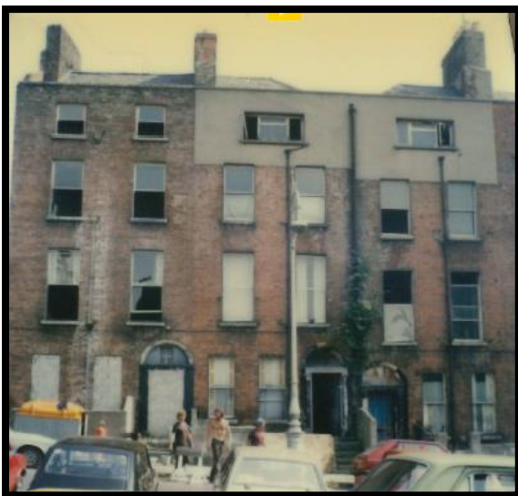
Figure 9 - View of structures no's 32-34 North Great George's Street circa 1983
