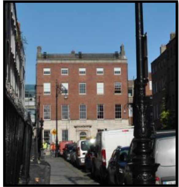
Figure 72 - Belvedere House, Denmark Street Great – landmark structure
