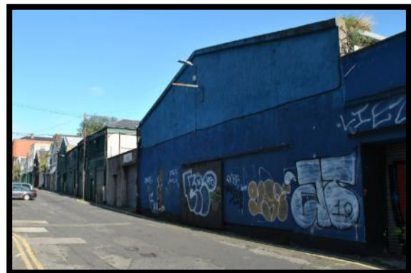
Figure 30 – The mews lanes streetscape Rutland Place
