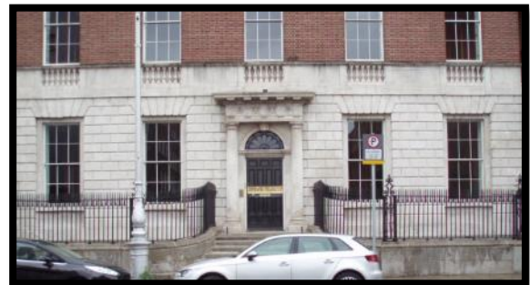
Figure 51 - Belvedere College – use of stone to ground level frontage
