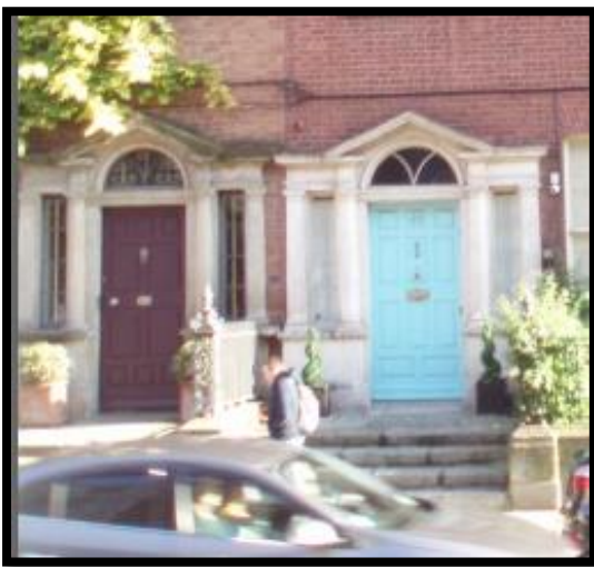
Figure 27: Nos 48 & 49 North Great Georges Street – matching stone door surrounds with the use of the Tuscan order
