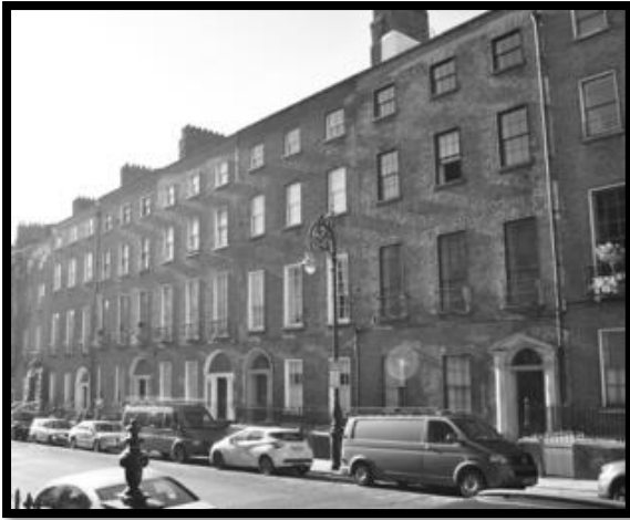
Fig 53 – North Great George’s Street – Typical 18th Century terraced roofscape – pitch roof concealed behind uniform stone parapet
