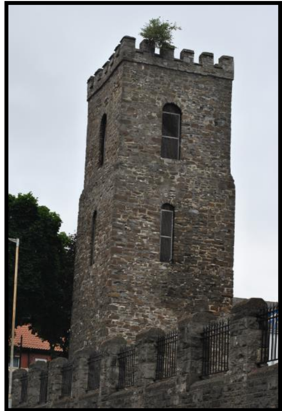
Figure 23 – St. George's Tower, Hill Street
