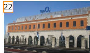
22 FORMER GOODS DEPOT - NORTH WALL QUAY (RPS 5843)
