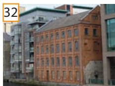
32 38-40 BARROW STREET (RPS 488)
