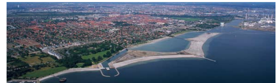
AMAGER STRAND, COPENHAGEN, A RECENTLY CONSTRUCTED ARTIFICIAL ISLAND
