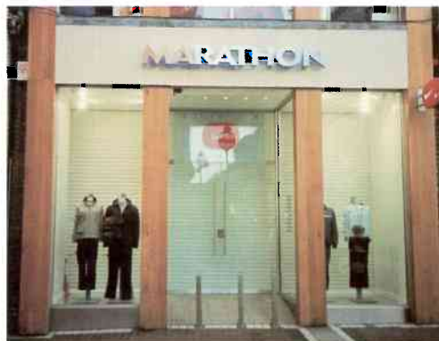
▼ Solid, heavy-gauge roller shutters set back behind the line of the window display allow for window-shopping after hours. An open-mesh shutter would be a further improvement.
