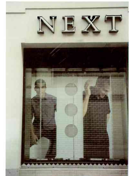
▲ Fine, open-mesh roller shutters on the inside face of the window allow a clear view of the shop's interior.
