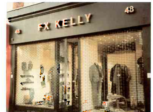
▼ Fine-gauge roller shutters set forward of the glazing allow the display to be seen after hours. Despite their slightness, a more elegant solution would be achieved if the shutter was located internally, behind the display area.
