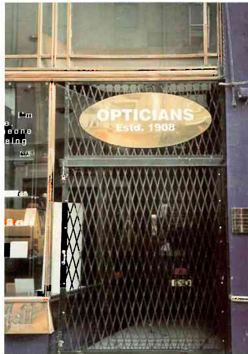
▲ A sliding open-mesh gate provides effective after-hours security for this recessed entrance.
