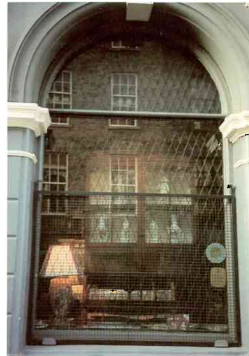
▲ A permanent, fine, open-mesh grille fitted to the inside face of the window, and a removable half-grille outside allow the window display to be seen clearly from the street.
