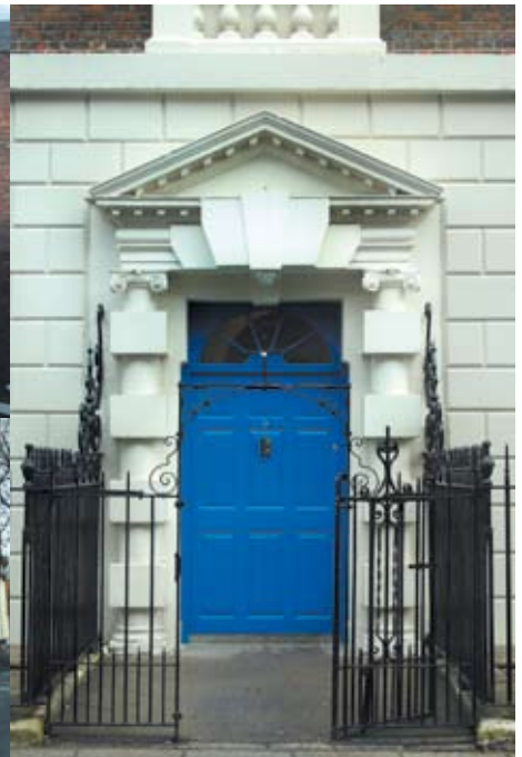
Fig.5.3.9 No.9, detail of doorcase
