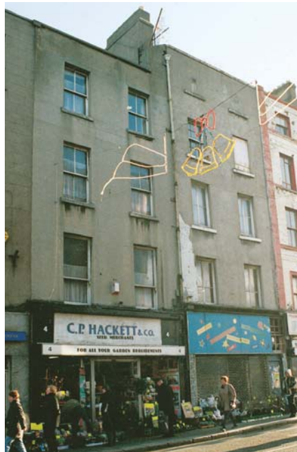
Nos 3 and 4 Capel Street before conservation works (left) and after (right). (The reuse of these buildings was a demonstration project for the 'Living Over the Shop' scheme by Dublin City Council).
