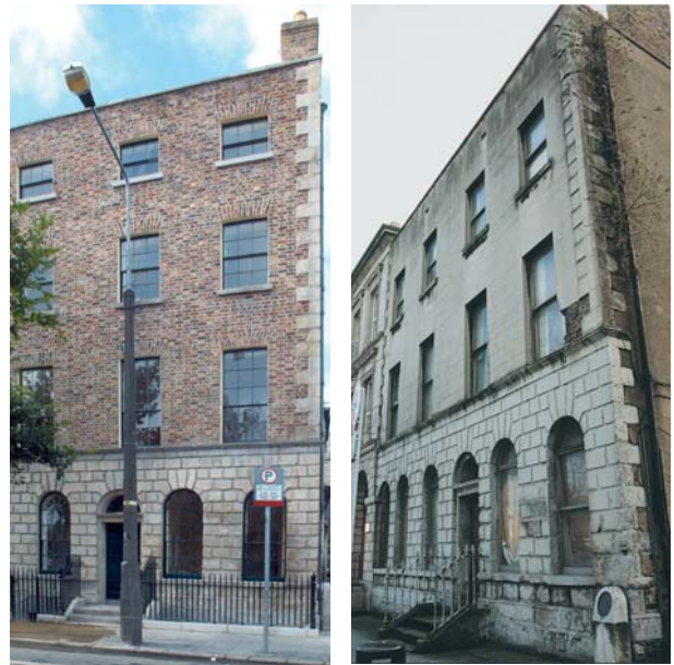
No. 9 Merchant's Quay before (left) and after conservation (right) which included the reinstatement of its third floor.
