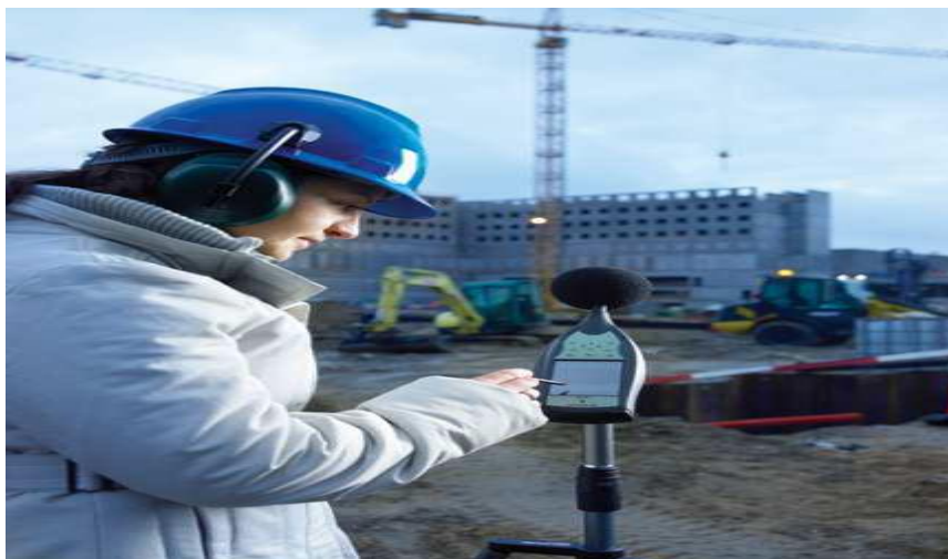
Figure 2: Noise Monitoring at a construction site (Source EPA)
