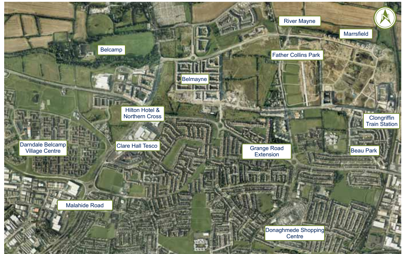
Fig 2.3 Aerial from 2009 showing the developing area of Clongriffin - Belmayne (North Fringe)
