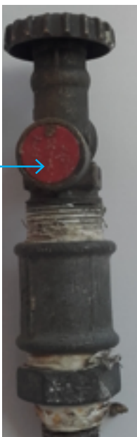
Photograph 8: Pressure relief valves and an emergency shut off
