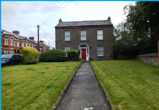
2 Belmont Avenue, protected structure
