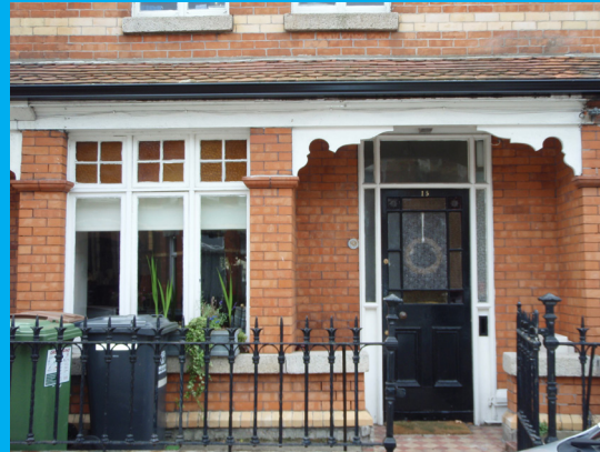
Ground floor detail of house at Belmont Park.
