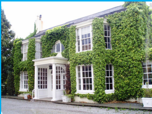
Belmont House, protected structure built circa 1720
