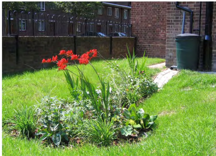
Photo above: rain garden in Ashby Grove, London (UK), here water is diverted from a downpipe. Designed by Bob Bray & Associates.
