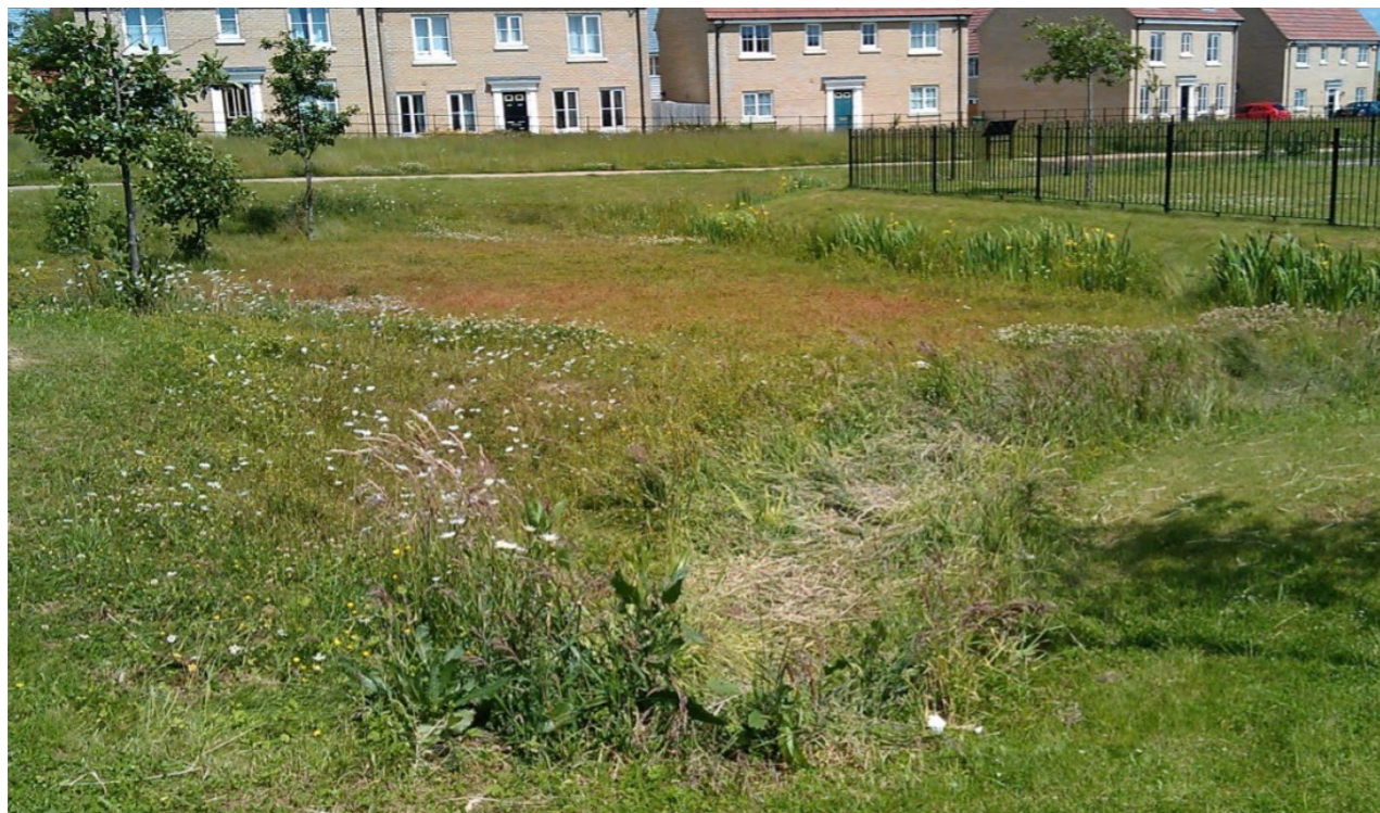
SuDS basin used for informal play by children. Basin has a low flow channel and majority of the basin remains dry for vast majority of the time.
