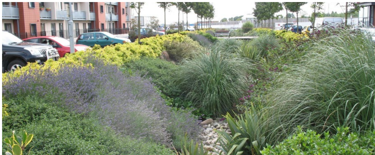
Image shows swale (linear basin) with potential for storing rainfall runoff (Pelletstown)
