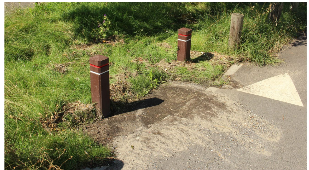
The gradual silt build-up at this kerb inlet into a swale was easily removed with a shovel.
