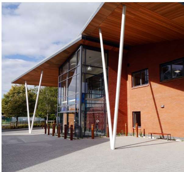
Image shows permeable pavement which stores flows within the sub-base using a flow control
