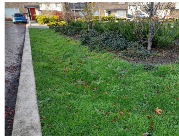
Collection of rainfall runoff using flush kerb and swale - Pelletstown
