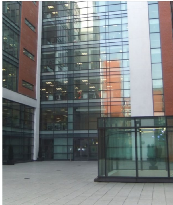
Permeable pavement courtyard constructed over a podium deck.
