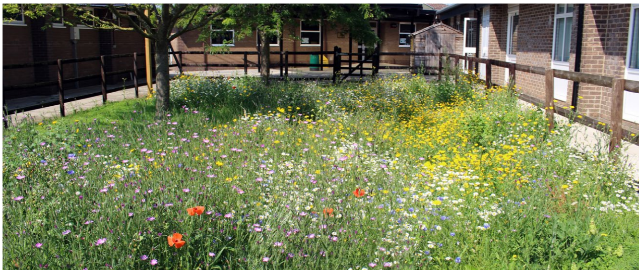
Example of a raingarden managing day-to-day rainfall (e.g. up to the 1 in 10 rainfall event) with flows passing onto subsequent features.
