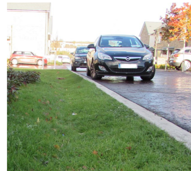
Low risk access road with sheet flow over a flush kerb and shallow conveyance swale. (Pelletstown)
