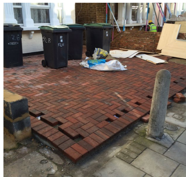
Paving front gardens is a common form of urban creep.
