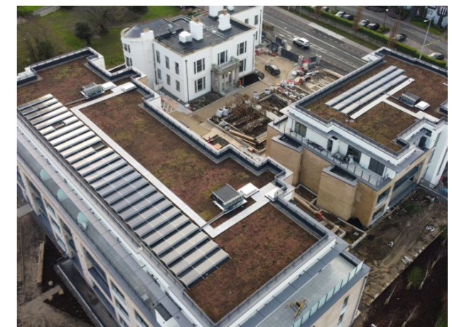
Green Roof Lower Kilmacud Road DLR
