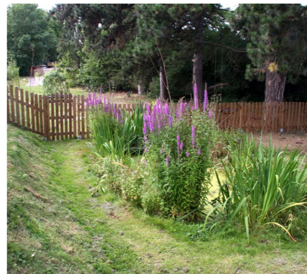
Example of a small wetland (with attenuation capacity over the permanent water level) located within a larger bunded grass attenuation basin.
