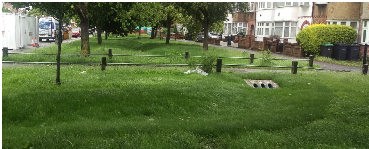
Image shows shallow short piped connection under a driveway allowing the swale to remain shallow downslope.
