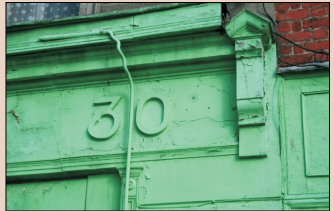
No. 30, Martin's Row, shop front detail
