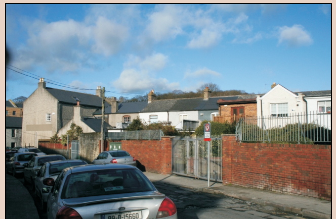
Rear of New Row: Note extensions
