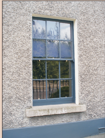
Timber sash window with early glass
