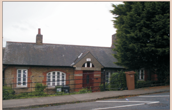
Chapelizod Hill cottage
