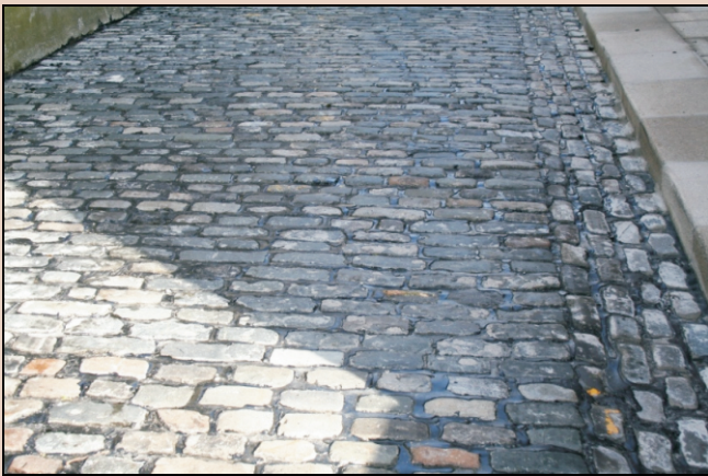
Recently refurbished sett-work to Chapel Lane
