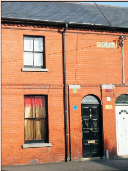
Brick-built dwelling, Liffey Terrace
