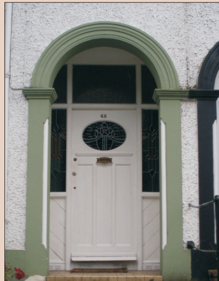
Timber panelled door in recessed porch
