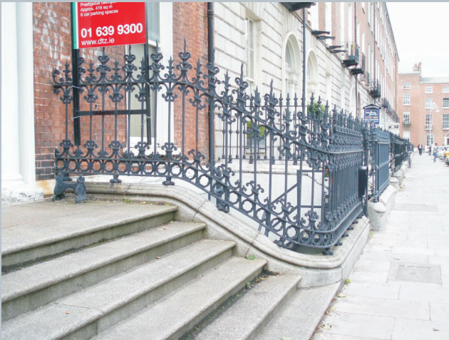
Photo 2.1.1 Georgian reinstated granite steps
