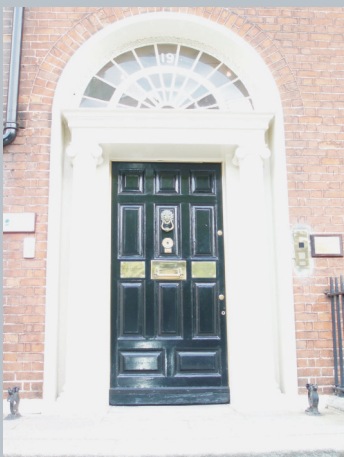
Photo 2.1.2.1 – Nos. 19 & 20 – Built by Henry, Mullins & McMahon. Included the firm's characteristic doorcase design in the form of flattened ionic capitals and fluted columns and feathered reveals on the windows. Robert Lloyd Praeger - The noted Irish naturalist lived at No. 19 between 1922-1952.
