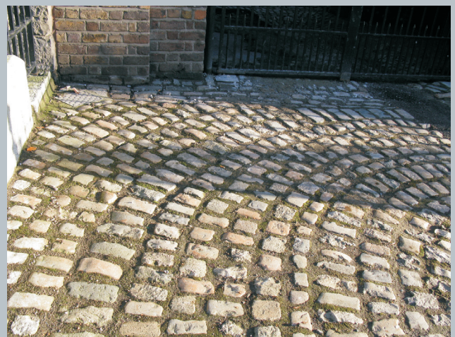
Photo 2.1.5.2 Decorative setts to carriage arch.
