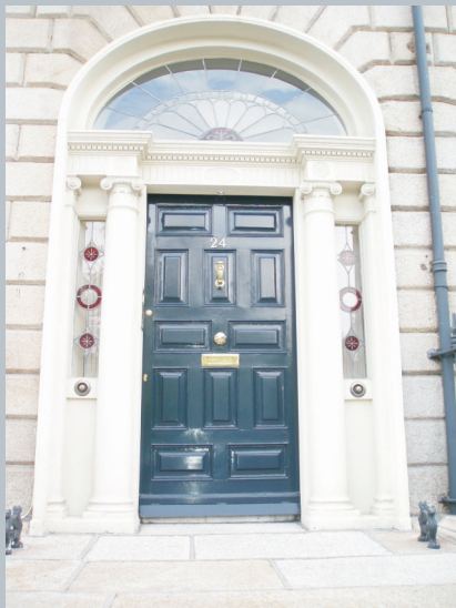
Photo 2.1.2.4 – Nos. 24 – 29 were built by Clement Codd. All six buildings have rusticated ground floors, extra long windows on the first floor and entrance doors with side lights as pictured above. No. 24 (pictured) is one of the few buildings that retains its intact mews house and garden.
