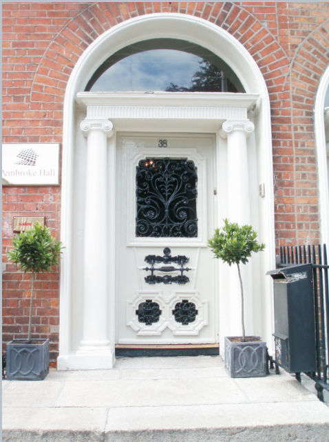
Photo 2.1.3.1 – Door of No. 38 Fitzwilliam Square
