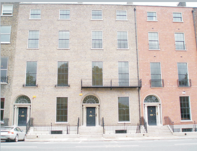
Photo 2.1.1.4 - Nos. 6-8 had a number of interventions that led to a loss of interior features due to the requirements of its change to commercial use in the latter half of the 20 th Century.
