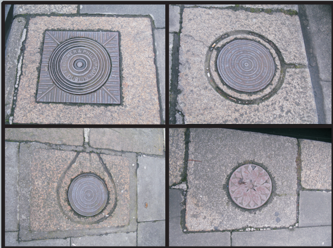
Photo 2.1.5.3 Examples of cast-iron coalhole covers in granite flags.
