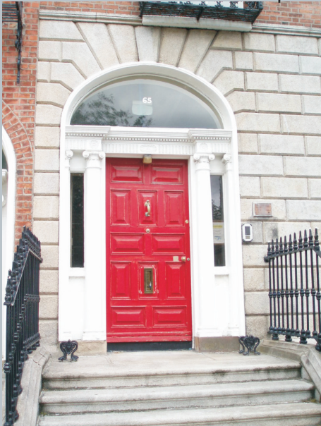
Photo 2.1.4.0 – Doorcase and original Granite steps to No. 65 Fitzwilliam Square
