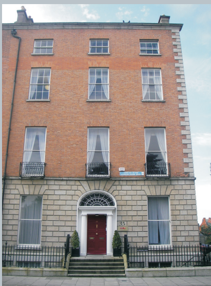
Photo 2.1.2.5 – Nos. 30-35 (No. 35 pictured) built by John Vance and this block is identifiable by the granite quoins at each end. All the doorcases and façade treatment are the same with Greek Doric doorcases.
