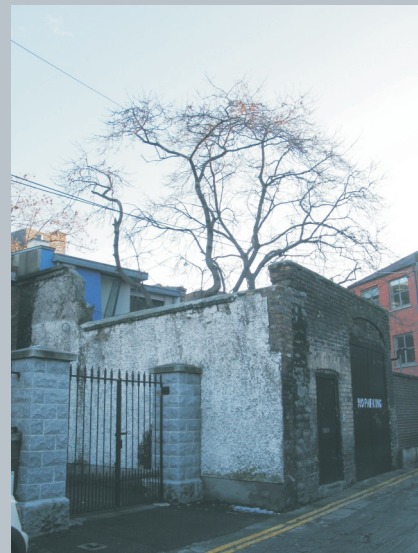
Photo 2.1.3.3 Yellow brick carriage arch
