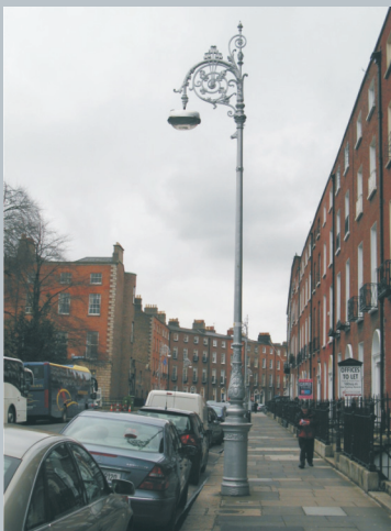
2.1.6.4 Cast-iron swan-necked street lamp.
