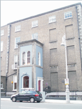
Photo 2.1.2.0 – No. 18 – Original windows and one bay only on the Square with the entrance on Fitzwilliam Place. It was built by Bernard Mullins and later associated with Jack B. Yeats.
