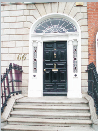
Photo 2.1.4.1 No. 66 Fitzwilliam Square displaying doorcase and long first floor windows.
