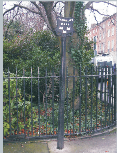
Photo 2.1.6.1 Original cast-iron ward sign with square profile railings to garden.
