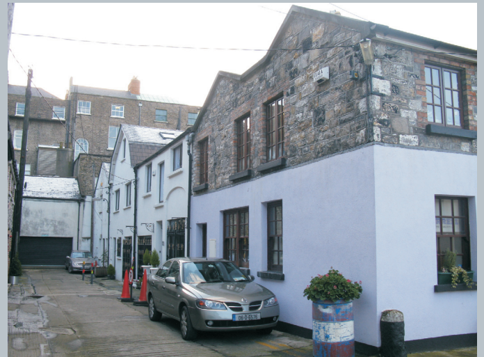
Photo 2.1.2.3 Rubblestone mews buildings
