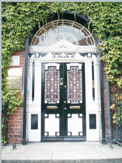
Photo 2.1.3.2 Door of No. 46 Fitzwilliam Square
