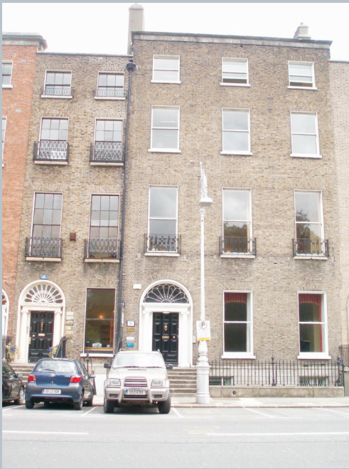
Photo 2.1.1.3 – Lord Fitzwilliam retained the plots of No. 4 and No. 5 until his death. No. 5 was neglected in the 1970s and lost most of its interior including its staircase. The façade was retained with the front facing rooms restored.
