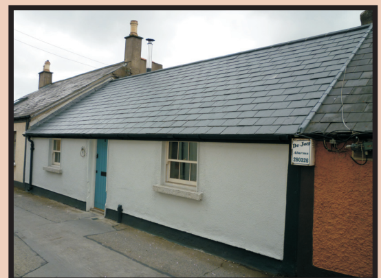
5 Westmoreland Park, newly renovated cottage with new granite sills, windows, newly rendered walls & natural slate roof.
