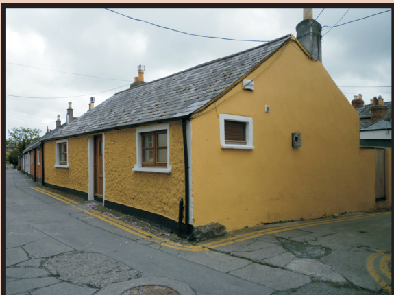
No. 4 Westmoreland Park, rough dash lime render intact.
