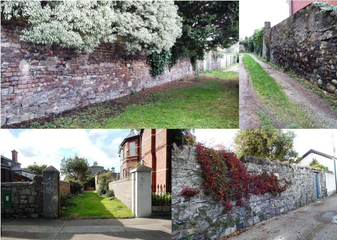
Clockwise from top left, view of section of surviving Clontarf Castle Demesne Wall composed of Brick and Calp Limestone to rear of 31-49 Victoria Road – section of wall shown is the rear boundary of 13 and 15 Kincora Road; view of Calp limestone wall along laneway adjacent to 51 Victoria Road; View of brick and granite wall in laneway between 1 Haddon Road and 92 Clontarf Road; view of surviving section of Calp limestone wall to rear of 37 and 38 Haddon Road.
