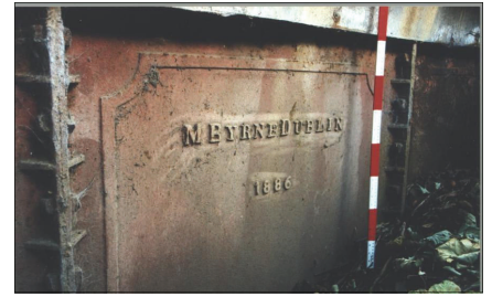
A panel of the cast-iron sectional aquaduct
