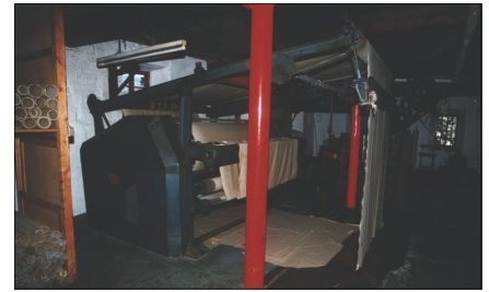
Brushing machine, Building 1
