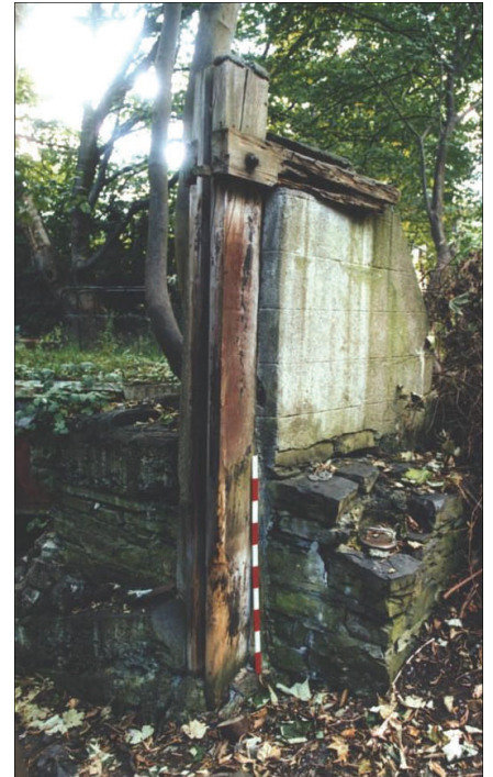
Surviving remnants of sluice gates
