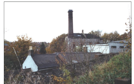
Kilmainham Mill from The Royal Hospital
