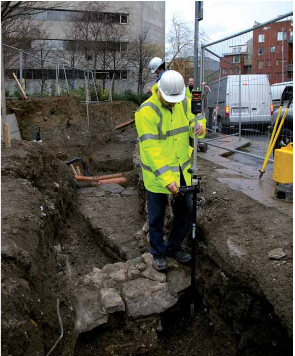
Fishamble St, Dublin 2 (Geodetic Survey & Laser Scanning Survey). Courtesy of MGL.
