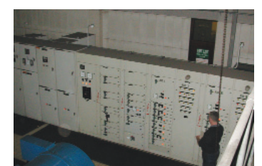
Electrical Services maintain the panels and switchgear for Water Services plant and for Drainage Services Pumping stations and equipment
