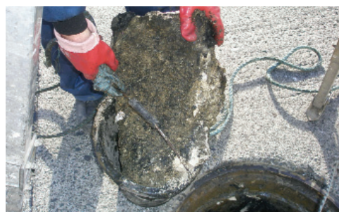
Blockage due to Fats, Oils and Greases - Georges Street
