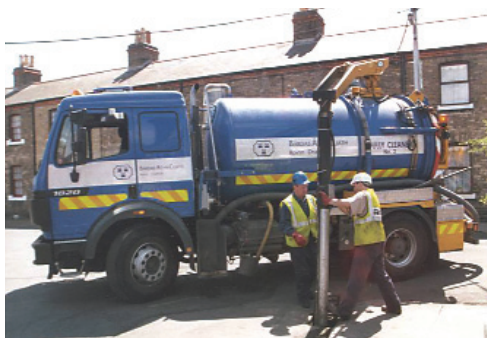
Gerry Fitzpatrick and Paul Dunne Gully Cleaning
