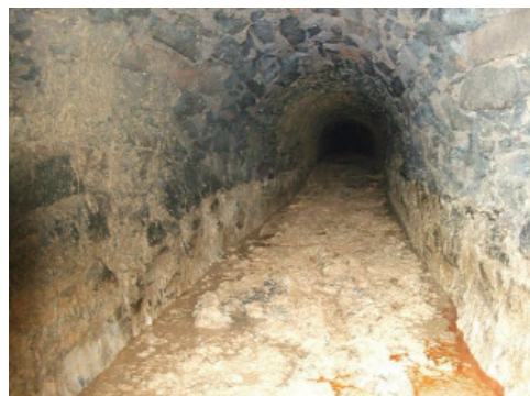
Blockage due to Fats, Oils and Greases - Georges Street
