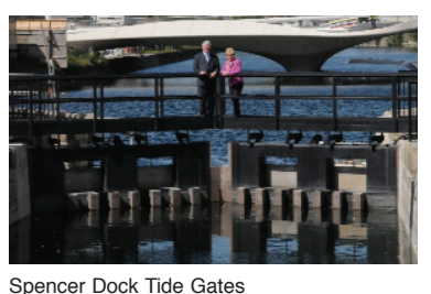
Spencer Dock Tide Gates
