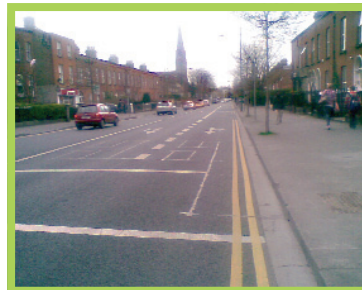
South Circular Road after resurfacing
