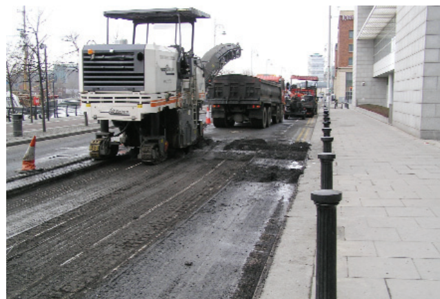
Reconstruction and overlay - Custom House Quay
