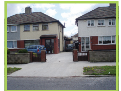
Shanliss Road footpath after repair
