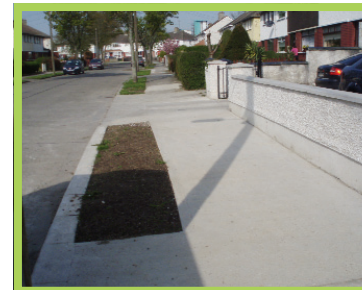
Oldtown Avenue footpath after repair
