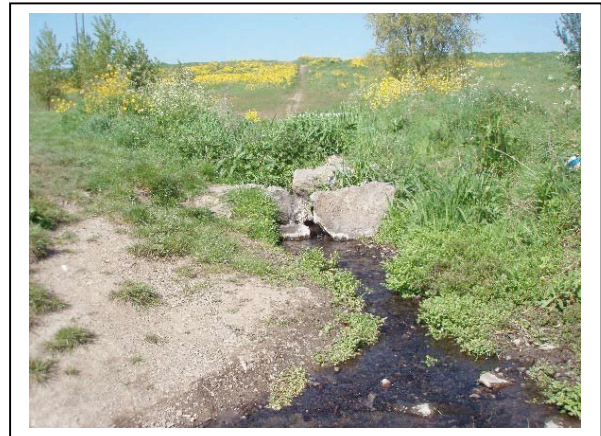
Discharge from Pond to River Tolka
