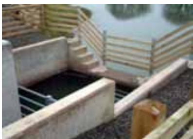
Concrete Lined Settlement Lagoon
