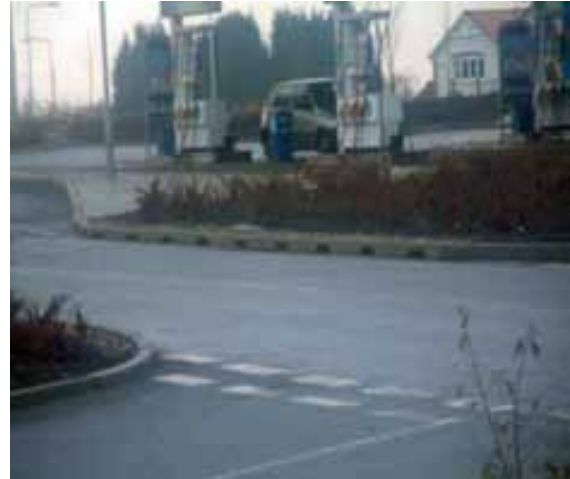
Side entry pits to filter drain filling station.
