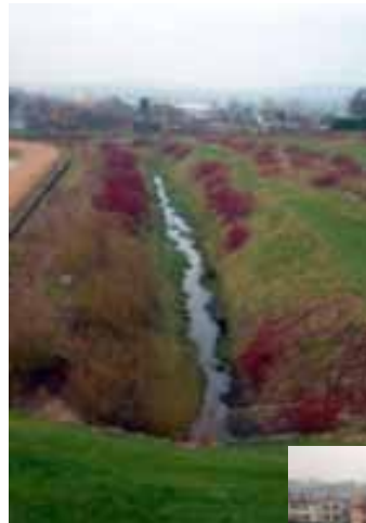
Large swale receives motorway drainage.
