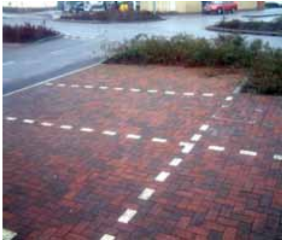
Permeable paving, "Tesco" carpark.
