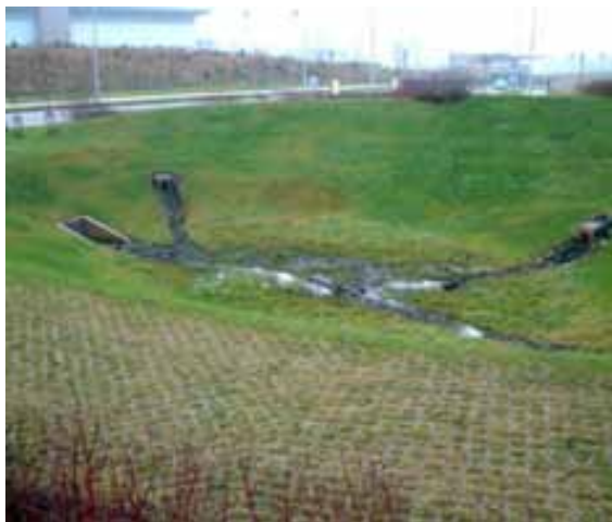
Detention basin makes use of space in roundabout. Grass-crete enables maintenance access.
