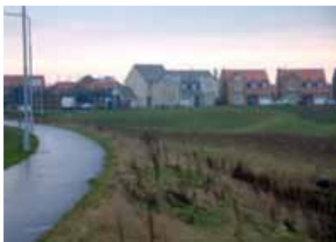
Large retarding basin and swale.
