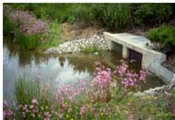
Outlet from loch provides outflow control.
