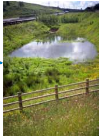
Settlement lagoons installed during construction; retained for permanent use.
