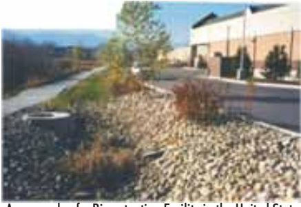
An example of a Bio-retention Facility in the United States
