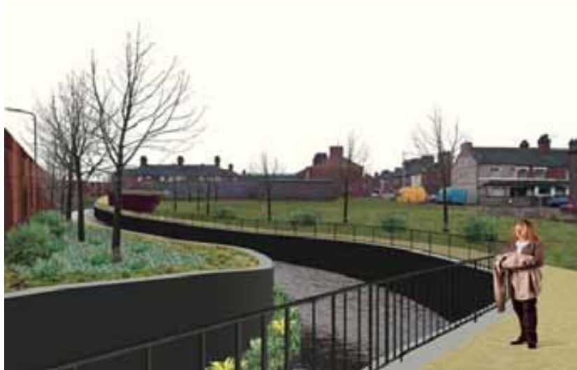
Figure 29: Realigned Channel with Meanders, Plant Benching, Pools and Riffles
