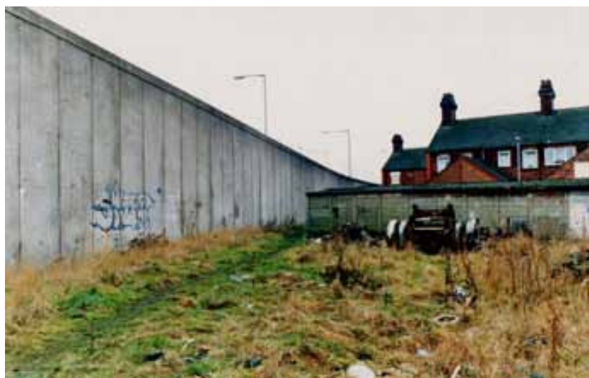
Figure 28: Urban Decay in Stoke before Culvert Realignment
