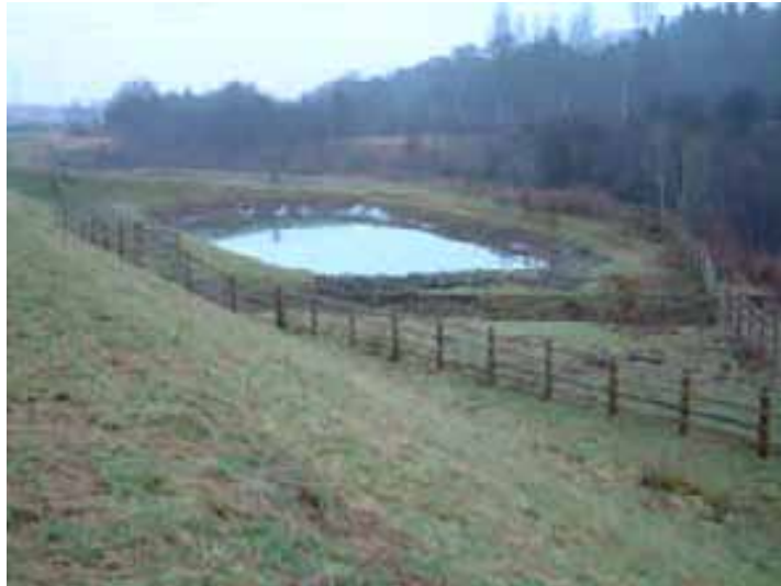
Figure 52: Roadside Retention Pond, Scotland
