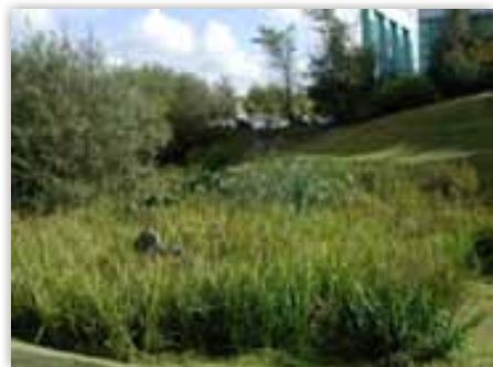
Vegetated Detention Basin
