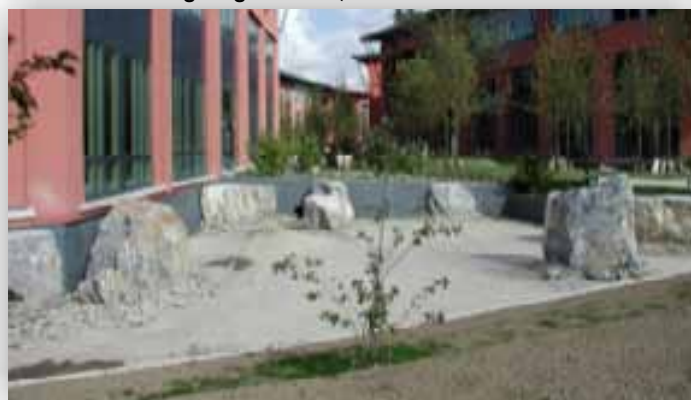
Dry Detention Basin, South Dublin
