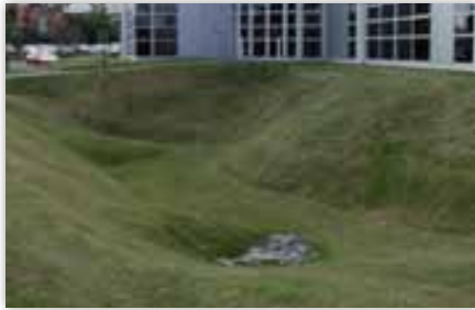
Grassed Detention Basin, South Dublin
