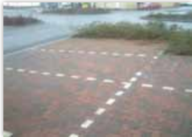
Traditional road surface drain permeable parking bays
