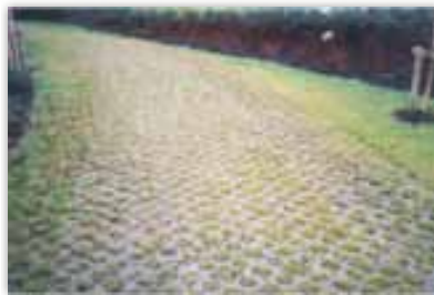
A "GRASSCRETE" Access Road in the U.K.
